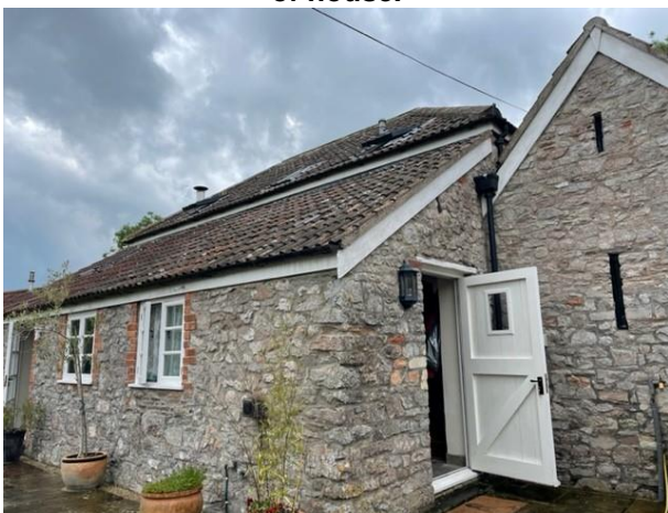
Photograph 3: Western elevation of house, roof void highlighted.
