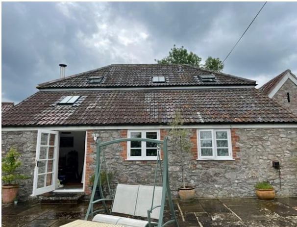
Photograph 1: View of northern elevation (rear) of house.
