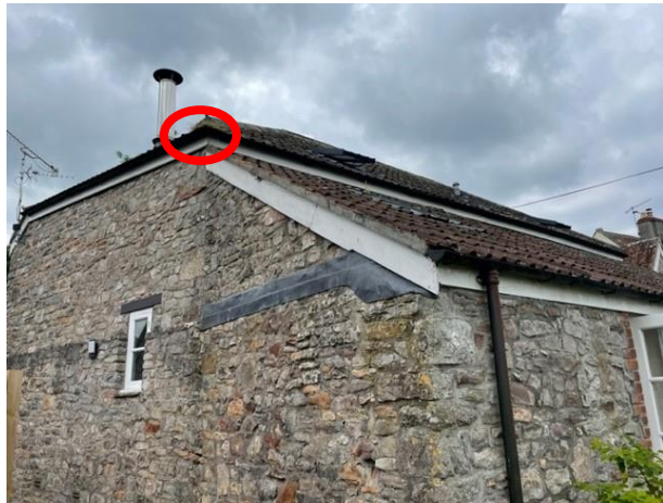
Photograph 2: Location of common pipistrelle emergence on eastern elevation.
