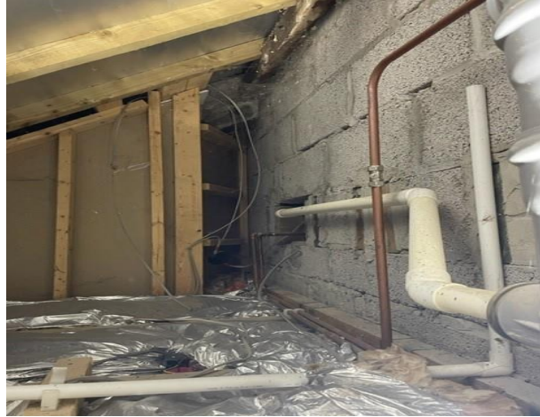
Photograph 8: View of roof void.
