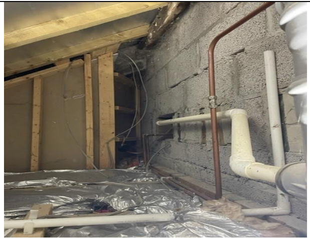
Photograph 8: View of roof void.
