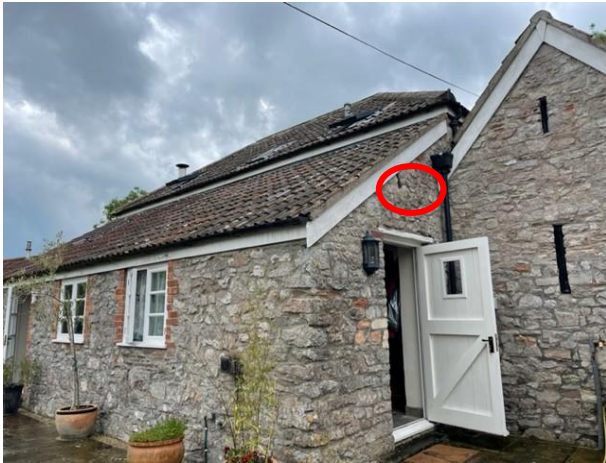
Photograph 3: Western elevation of house, roof void highlighted.
