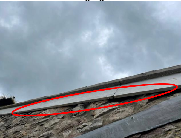
Photograph 5: Example of roosting feature under fascia boarding.
