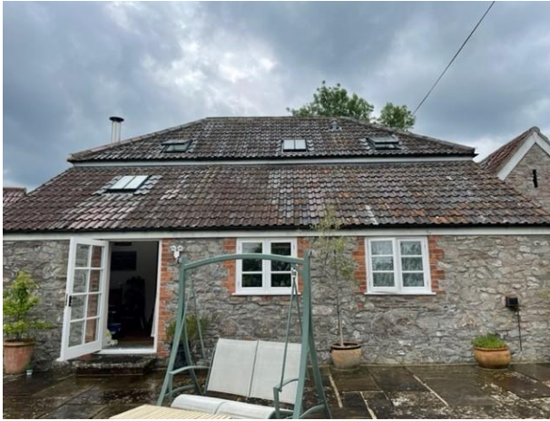
Photograph 1: View of northern elevation (rear) of house.
