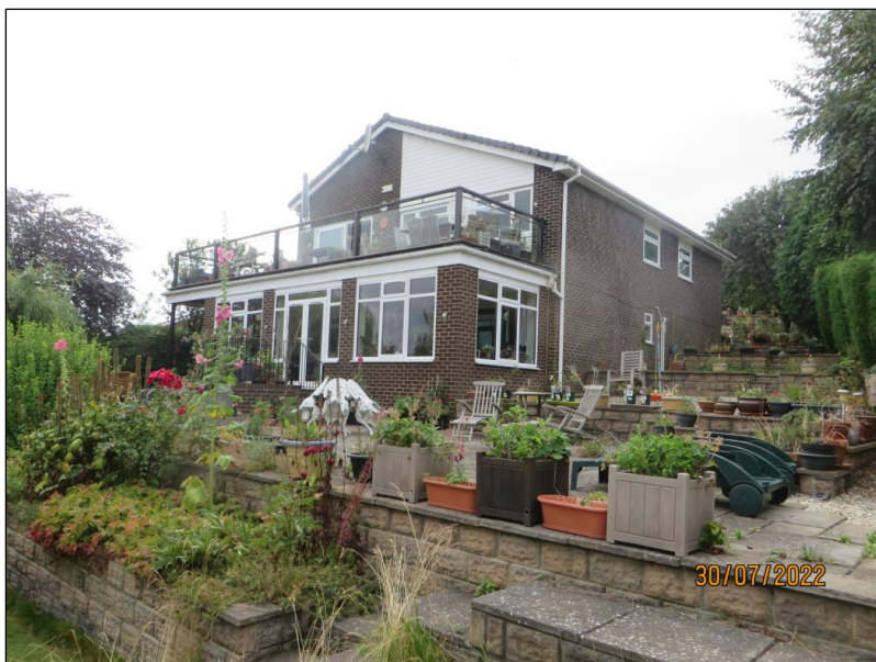
Figure 9. Rear (south eastern) and side (north eastern) elevations.
