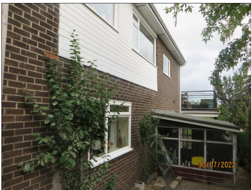
Figure 11. South western elevation showing wooden porch area.
