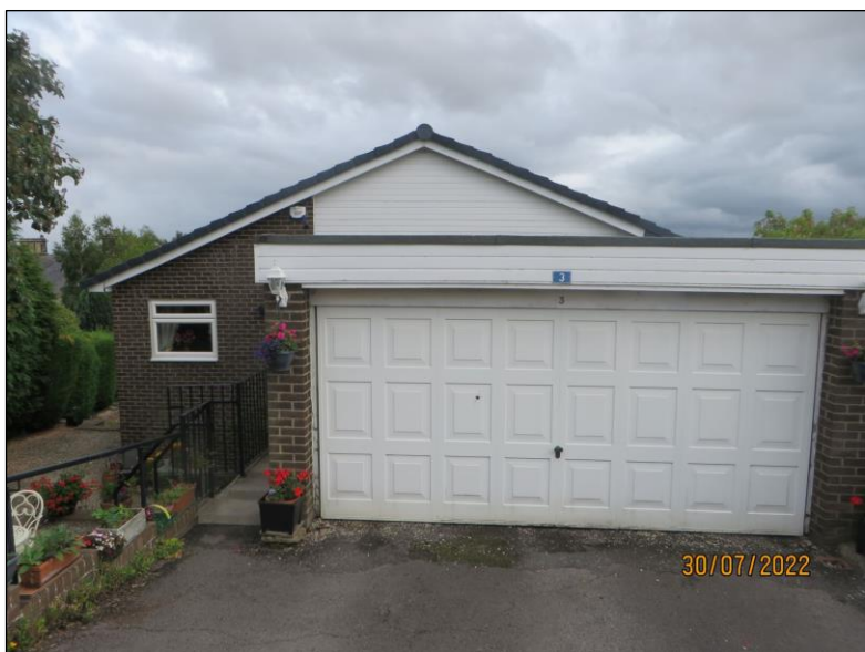
Figure 10. Front (north western) elevation.
