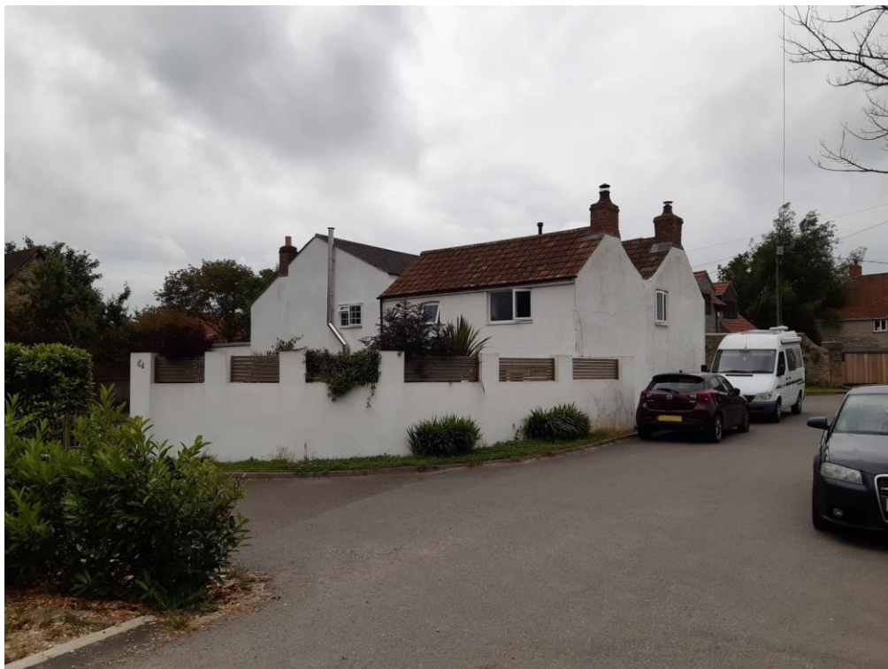
North East Elevation and North West from the street view.
