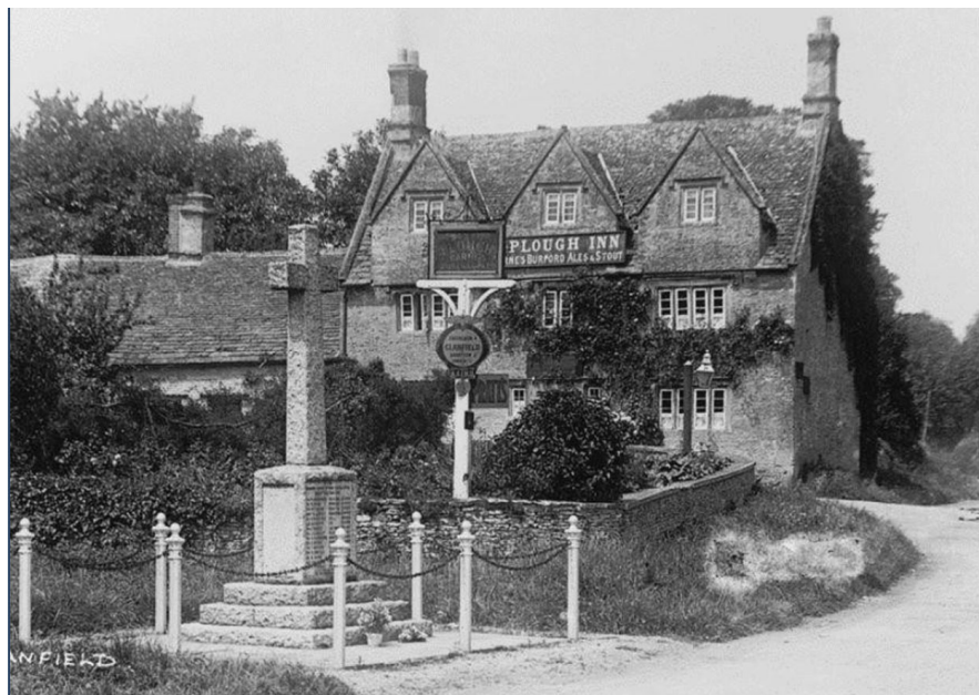
Figure 4. A photograph of the Site taken c.1920s showing the mid-17 th century three bay range with the 19 th century single storey infill extension projecting to the left. The Site changed use from private residential use to public house sometime in the 19 th Century.
