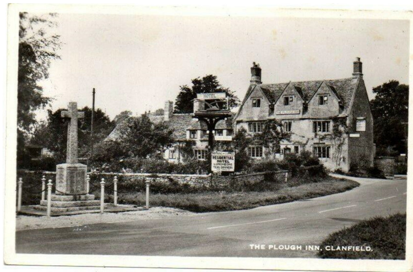
Figure 3. A postcard from the 1960s showing the Site with minor alterations to the plan form, including the construction of dormer windows to the 19 th century western infill extension
