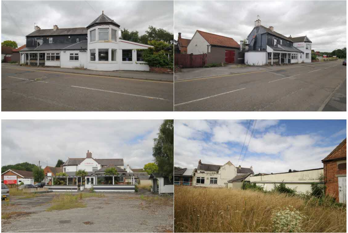
Plate 13: Exterior of the former pub.
