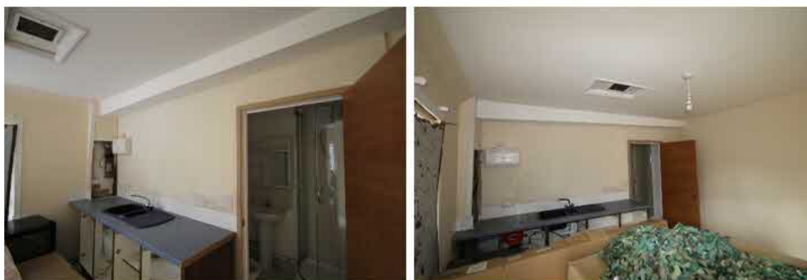
Plate 19: The middle section of Outbuilding A and its interior.
