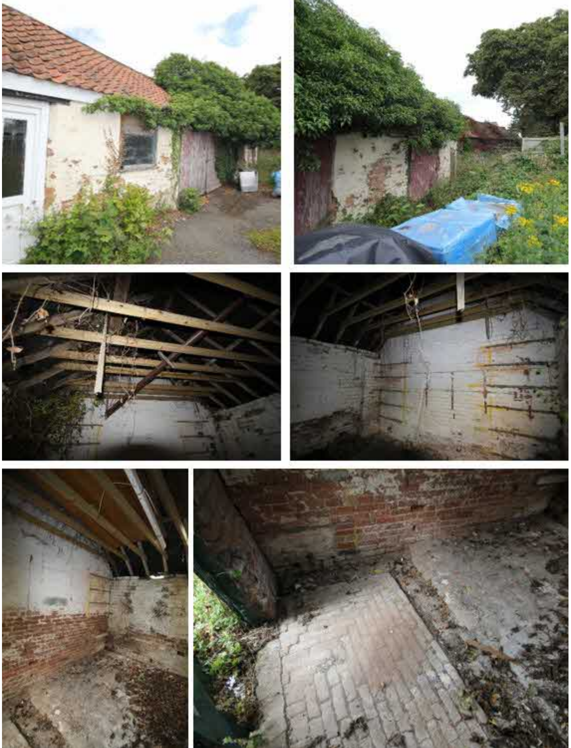
Plate 20: The end third of Outbuilding A and its interior.
