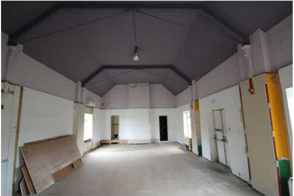
Plate 22: The front, rear, and interior of Outbuilding B.
