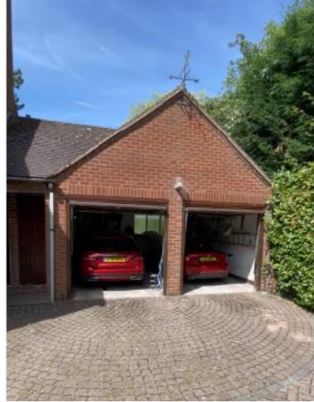
Garage to be removed and reduced in width to make way for extension
