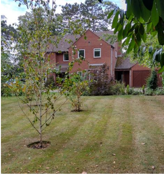
Frontage of existing house with garage to right
