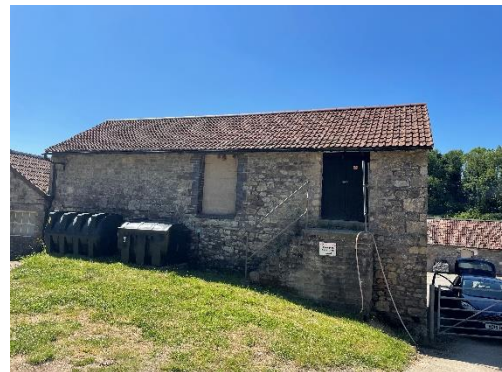
Plate 2: Barn (Northern Aspect)
