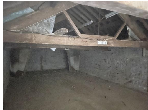
Plate 6: Barn – Interior (Upper-floor)
