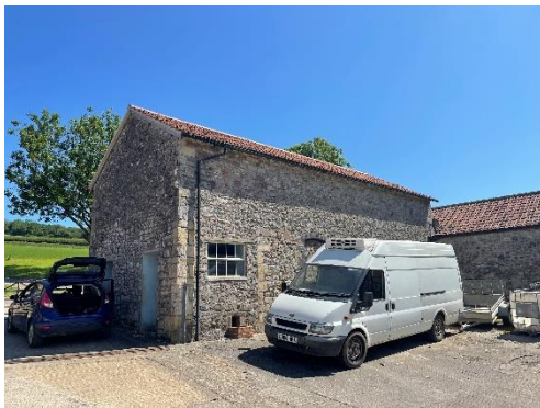
Plate 1: Barn (Southern Aspect)
