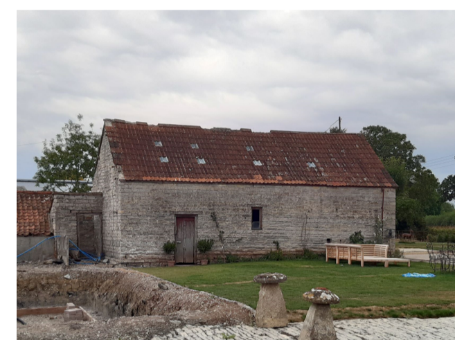
Site Photo 01. Existing West elevation of Barn 3 viewed from courtyard.
