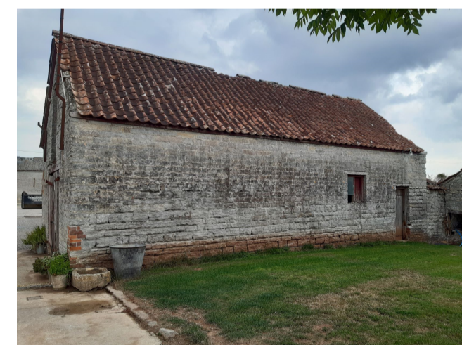
Site Photo 03. Existing East elevations of Barn 3 viewed from driveway.
