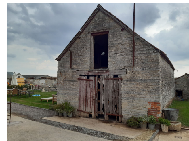
Site Photo 02. Existing South elevation of Barn 3 viewed from driveway.
