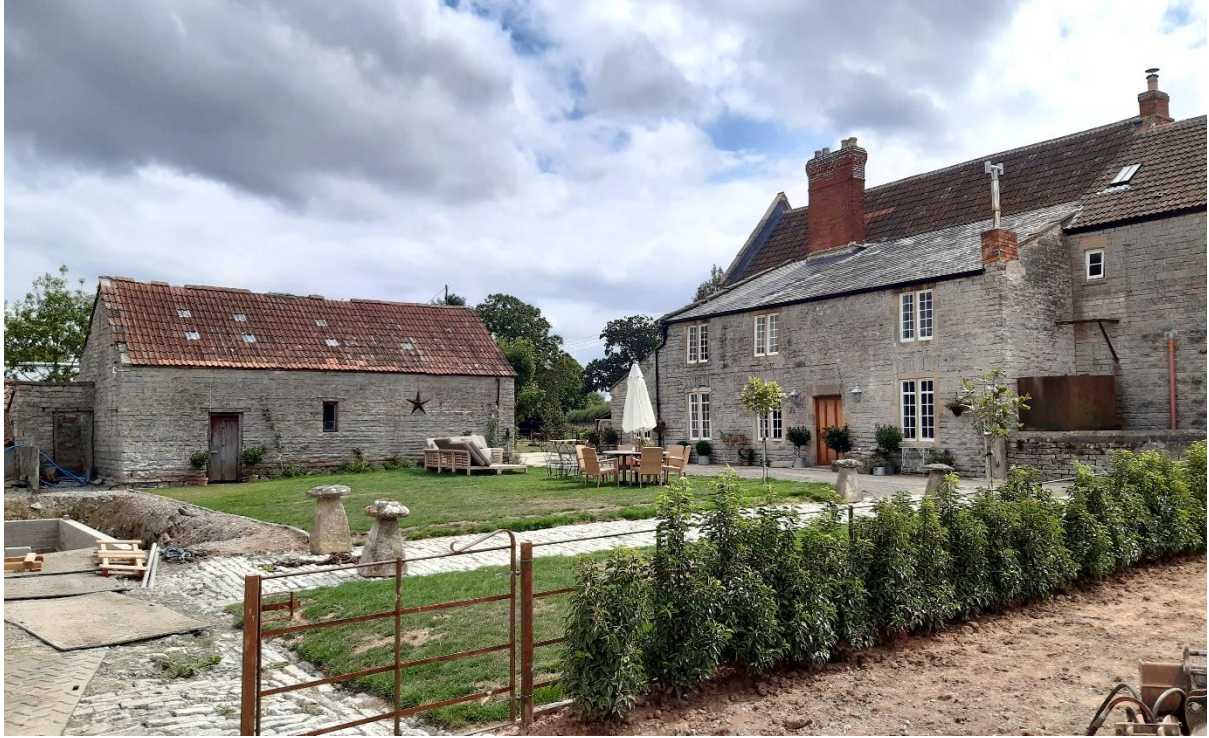
Image 2 – Rear (north) elevation of Manor Farmhouse and west elevation of adjacent barn viewed from courtyard.
