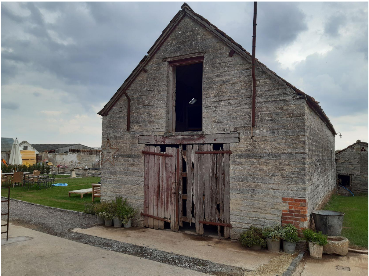
Image 3 – South (end) elevation of barn viewed from driveway.
