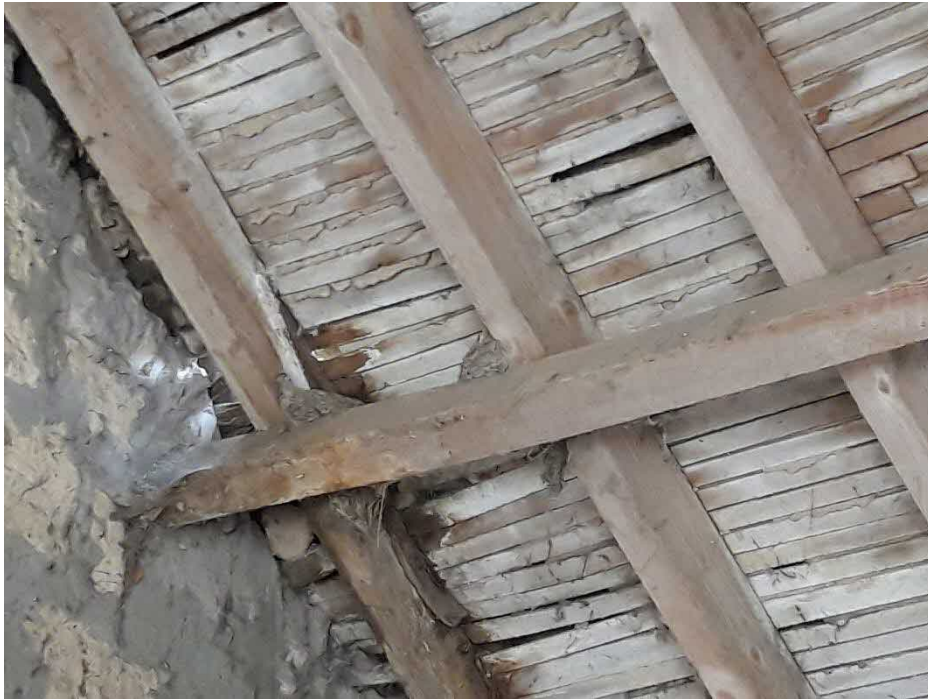
Photograph 1 – Interior of former stable/cart shed
