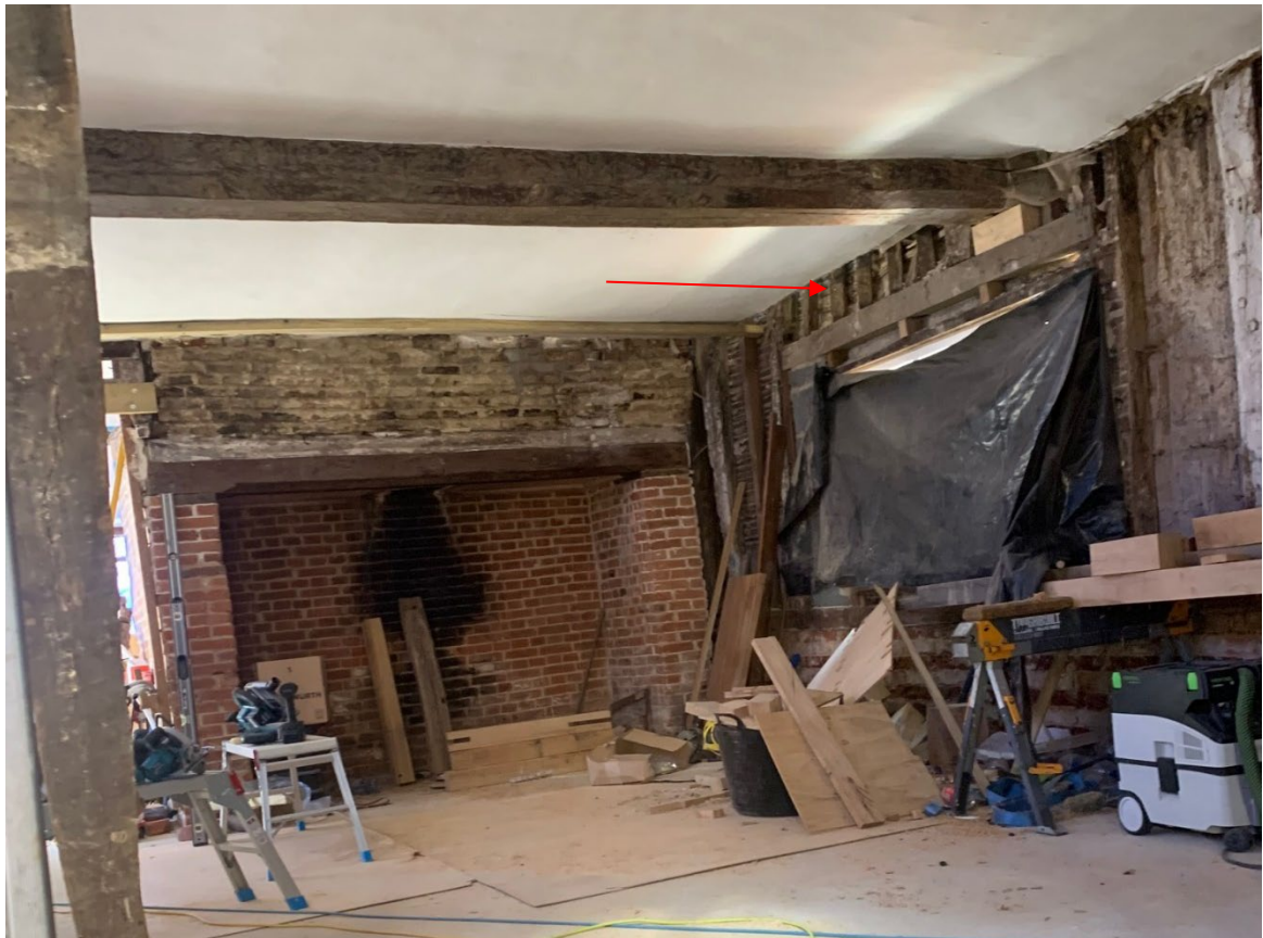
Figure 5: 2-Bay Hall with part surviving diamond-mullioned windows.
