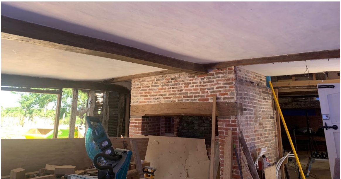
Figure 14: Ground Floor Parlour and fireplace.
