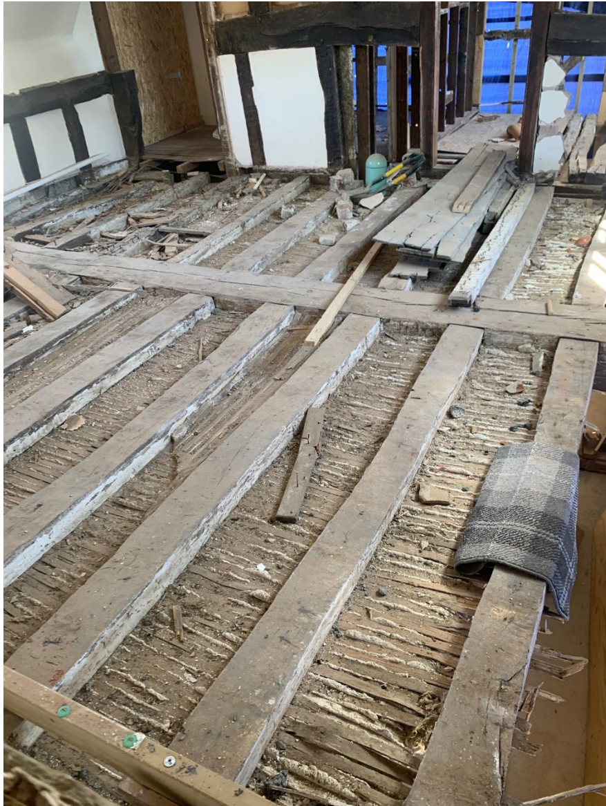
Figure 12: Inserted floor over the former open hall.
