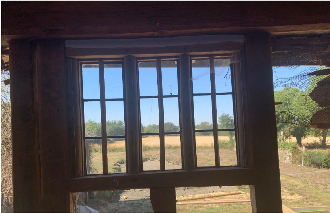
Figure 17: 3-Light ovolo-mullioned window in the parlour chamber.
