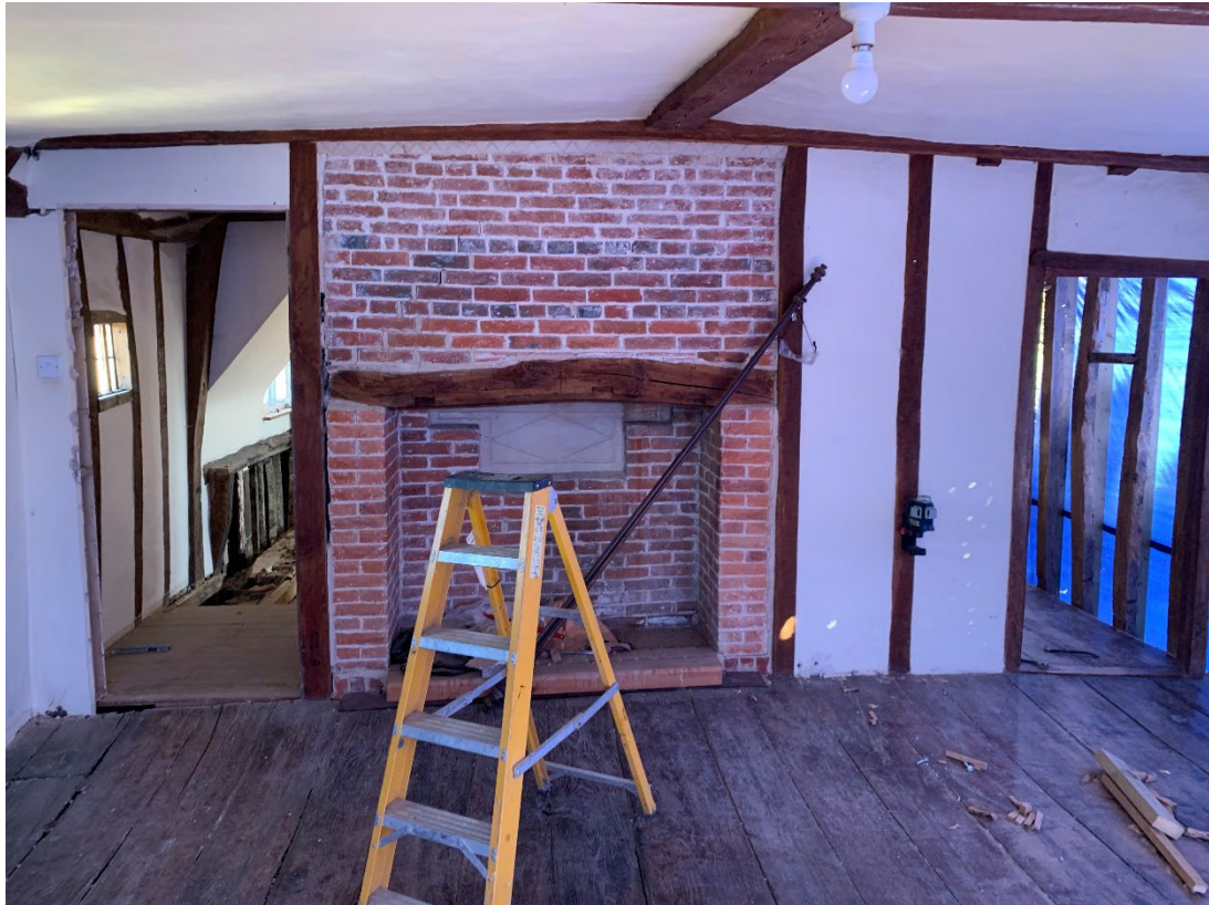
Figure 15: Parlour Chamber fireplace.
