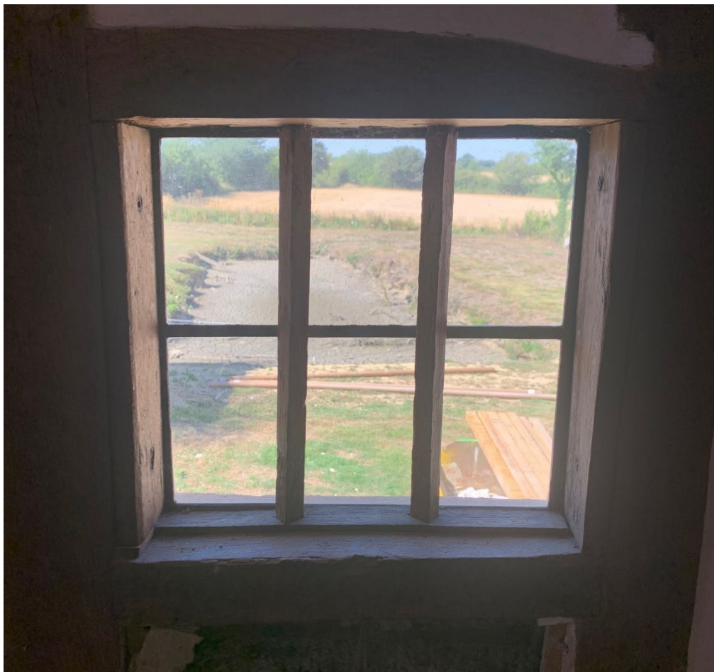
Figure 18: 3-Light 17 th century diamond-mullioned window in the first-floor 'chimney bay'.
