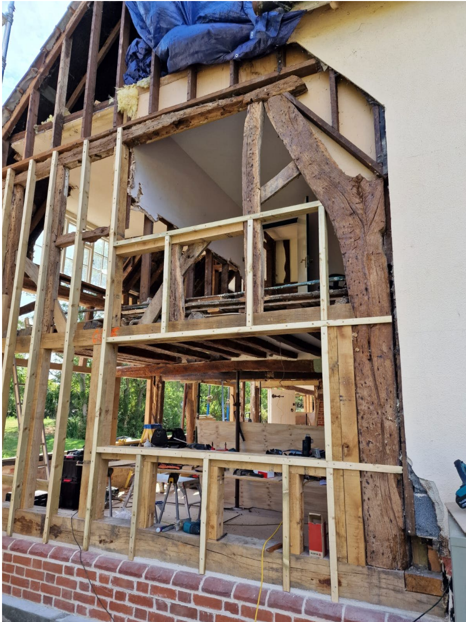
Figure 8: Base-Cruck construction to the north end wall
