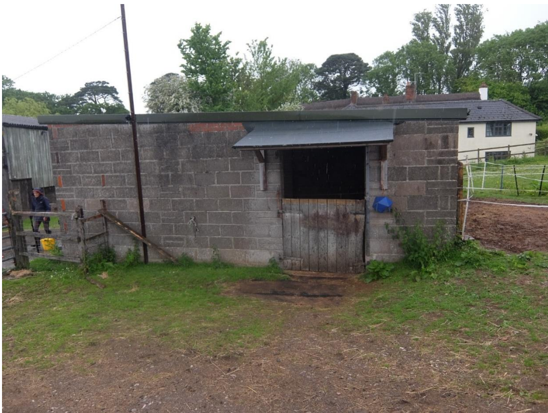
Right side wall
