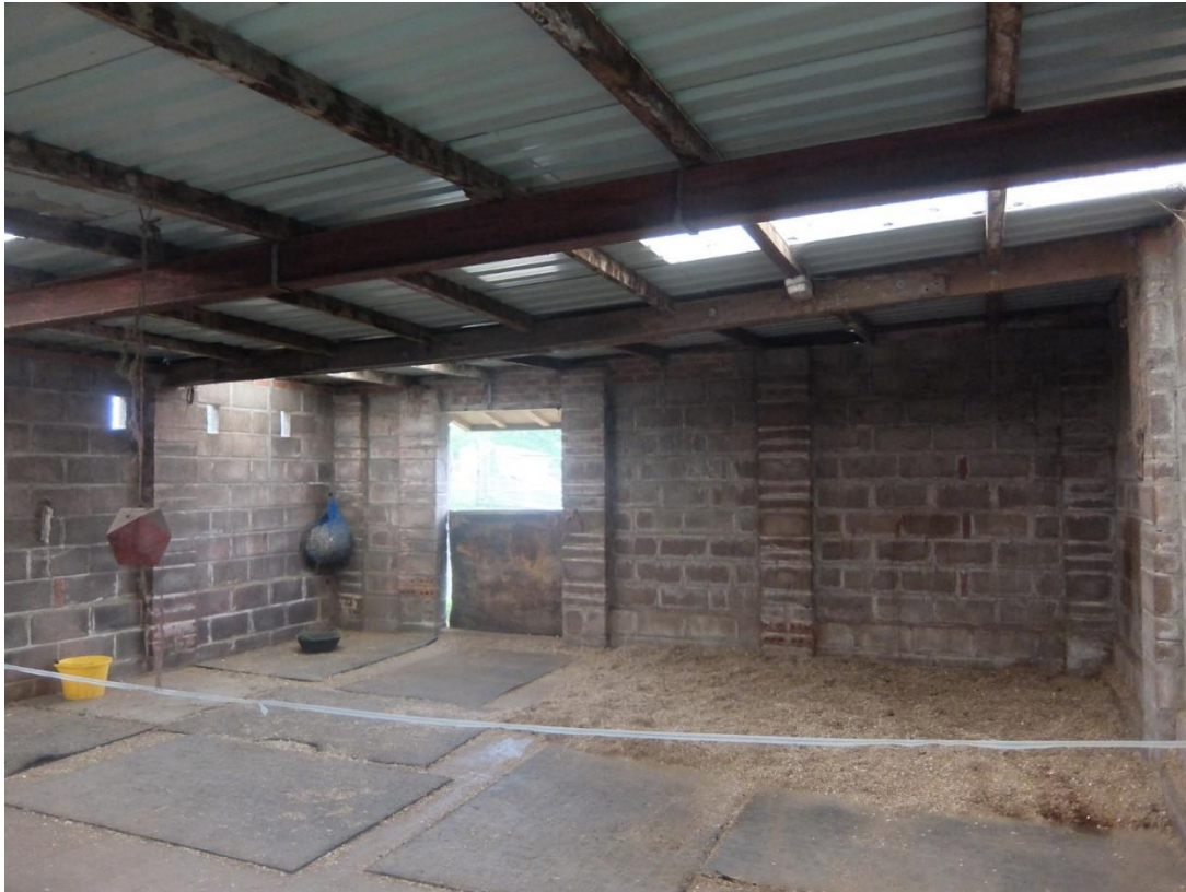
Internal view looking towards right side wall
