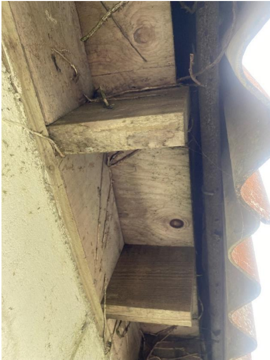
Figure 5: Gaps leading to the mezzanine floor and up behind the corrugated sheeting (left), and gaps underneath the roofing sheets and ridge tiles (right).
