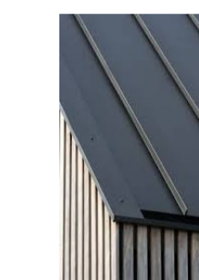
METAL STANDING SEAM ROOF
