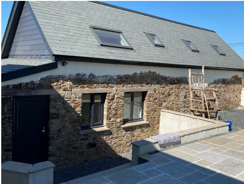
Photo of the existing building
