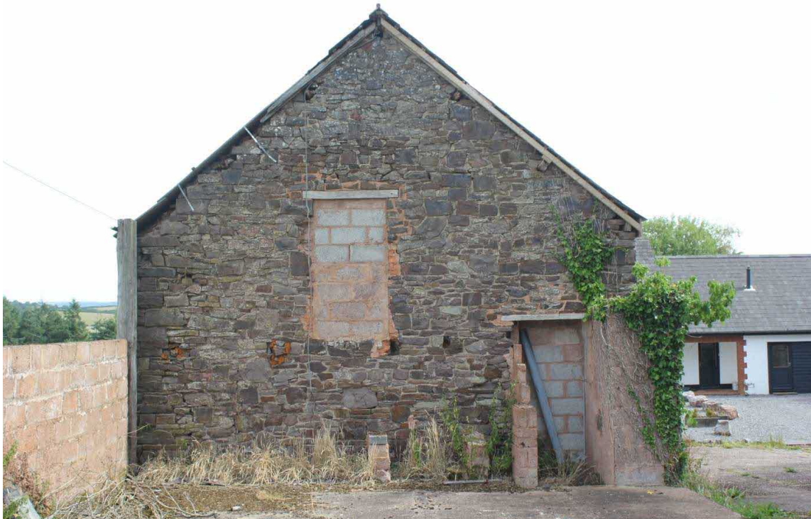
Photograph 4 Gable (South) Elevation
