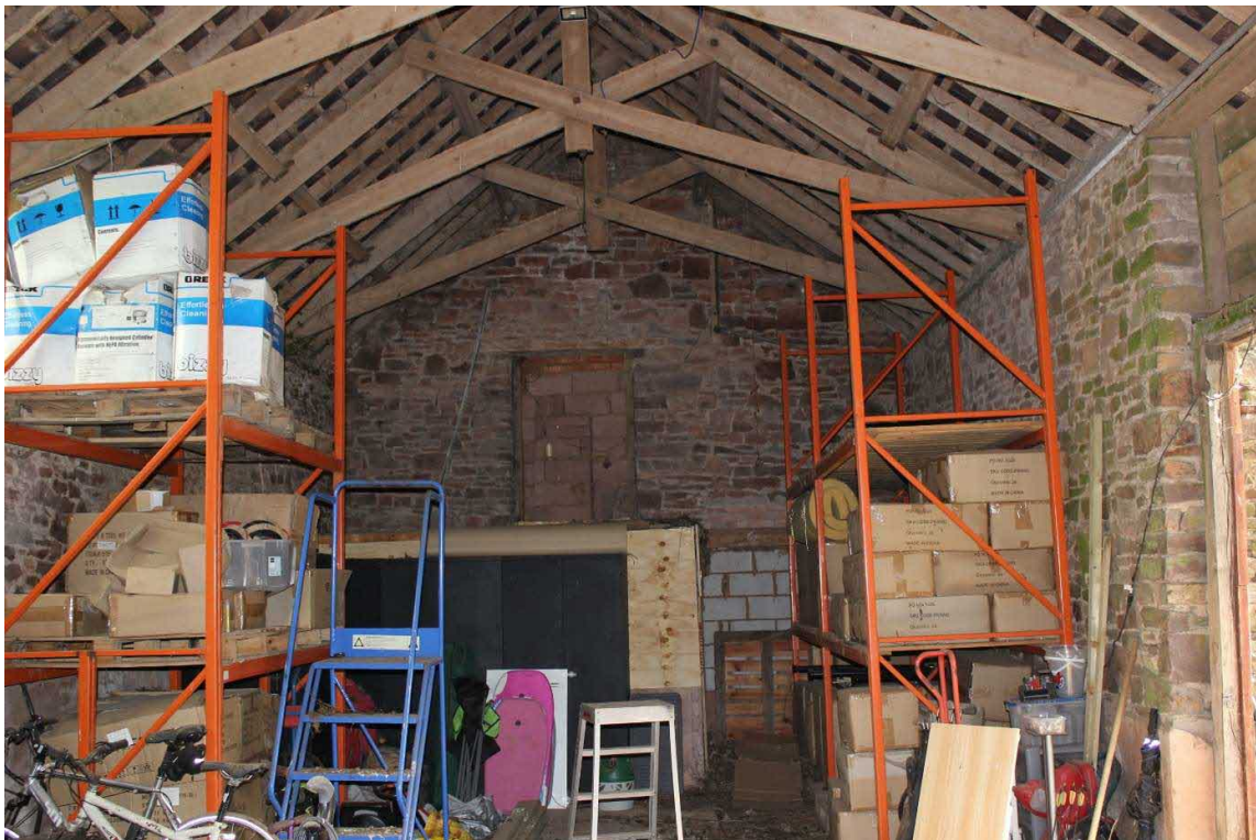
Photograph 8 Internal View Looking North
