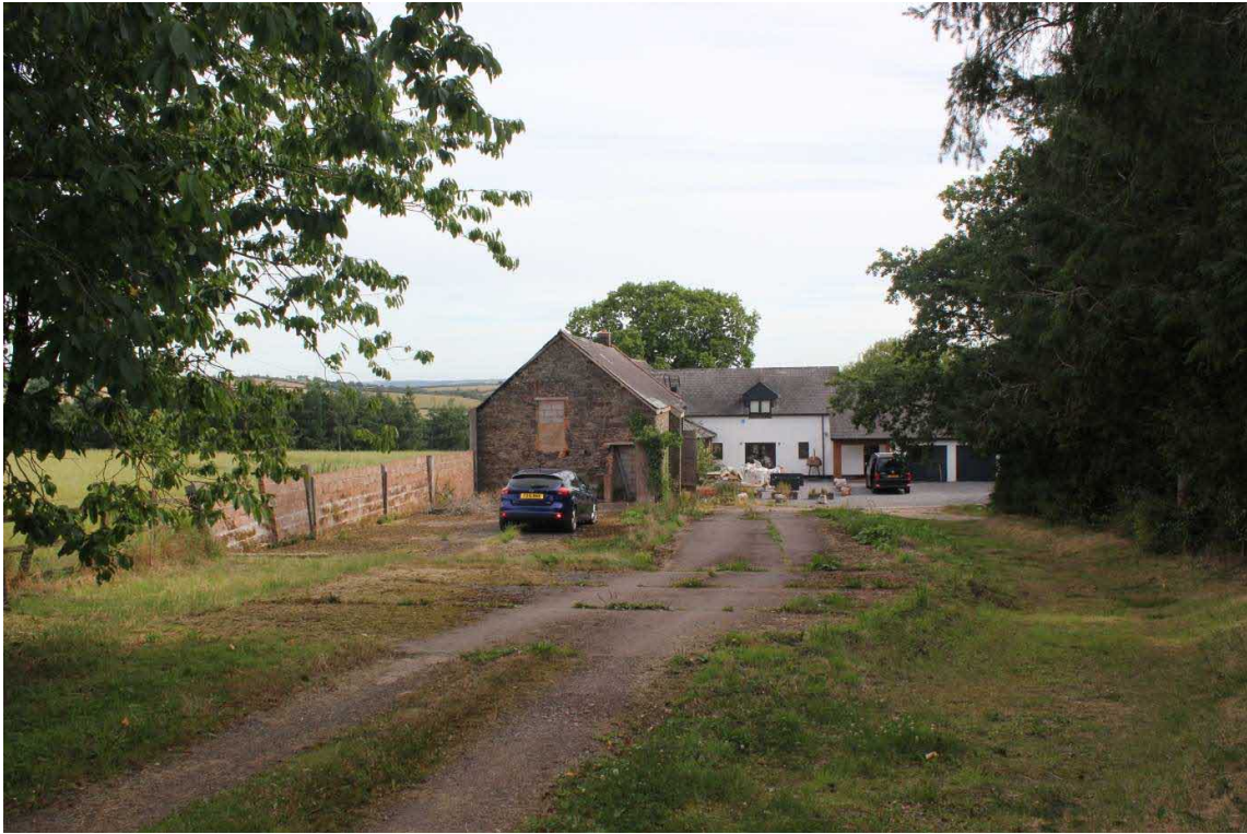
Photograph 1 View From Site Entrance
