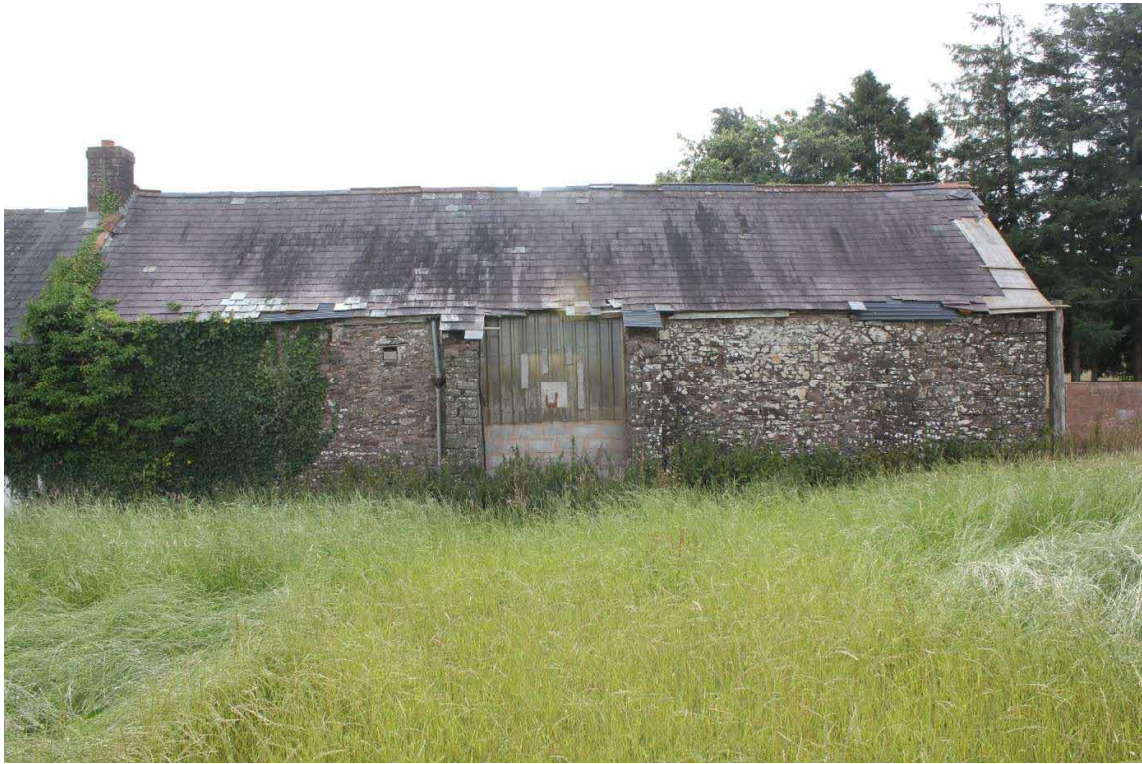
Photograph 5 Side (West) Elevation
