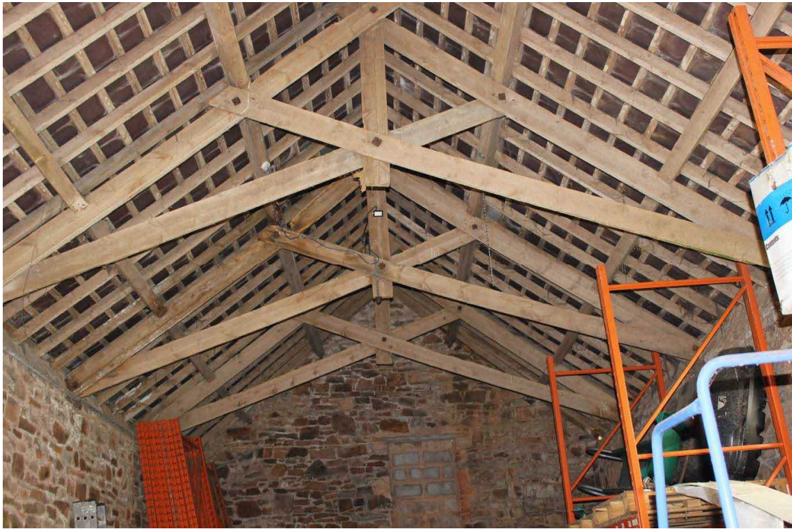
Photograph 9 Internal View of Roof
