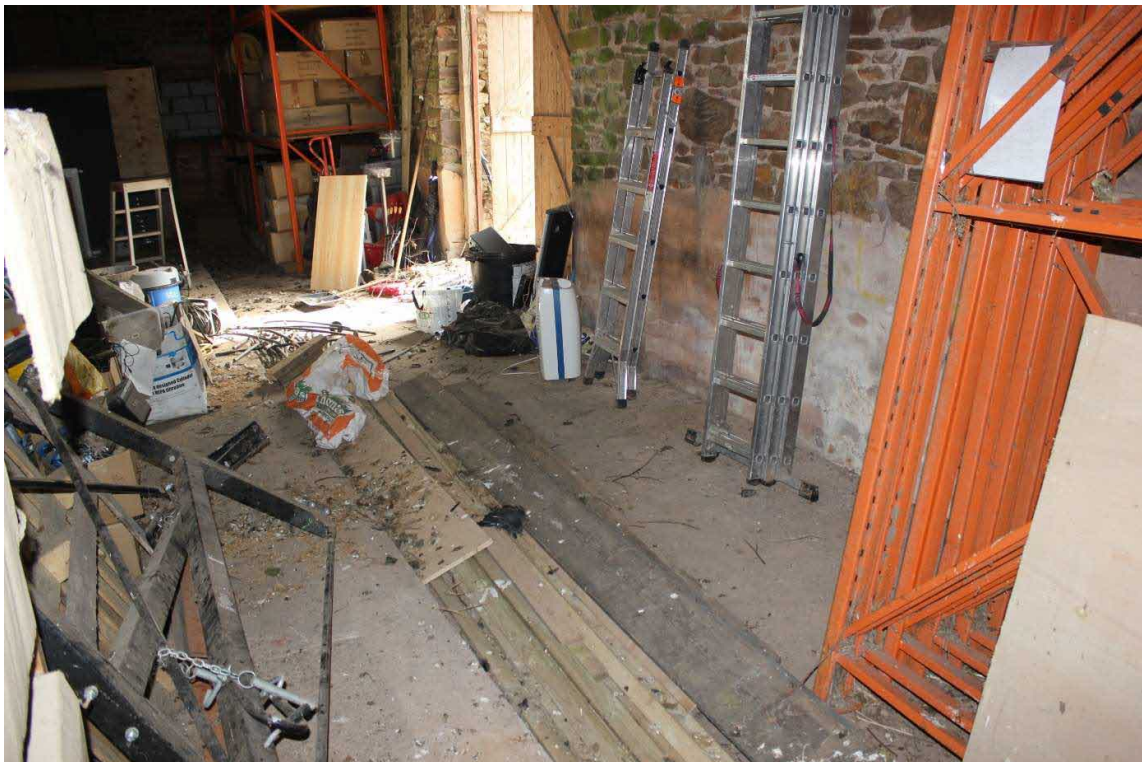
Photograph 10 Internal View of Floor
