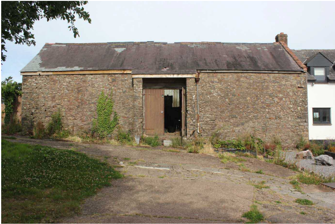
Photograph 3 Side (East) Elevation
