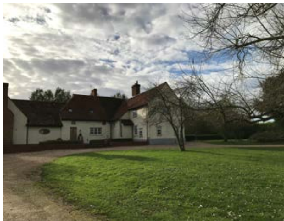
Figure 17 : Friars Farm, view of north elevation.
