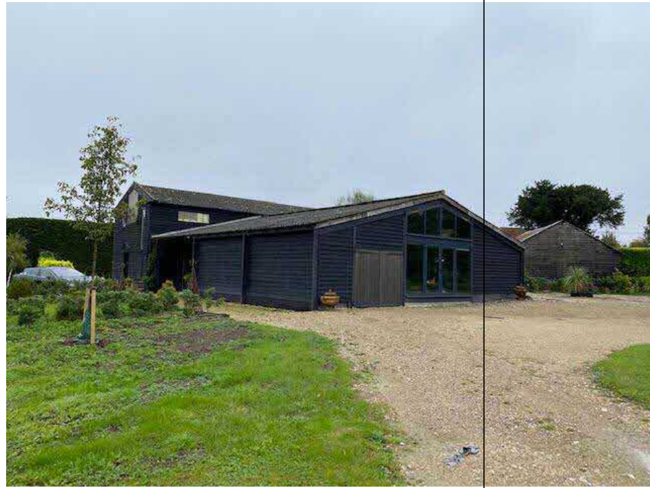
2. Converted agricultural storage building.
