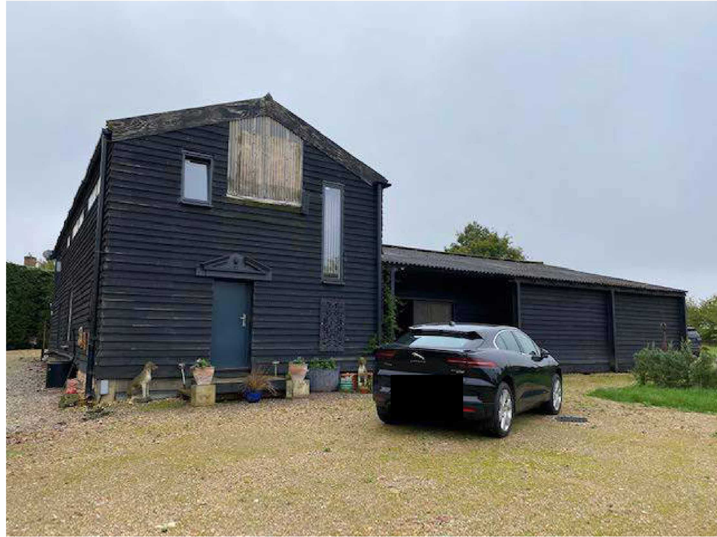
Outbuilding & Big Barn South Eastern Elevation
