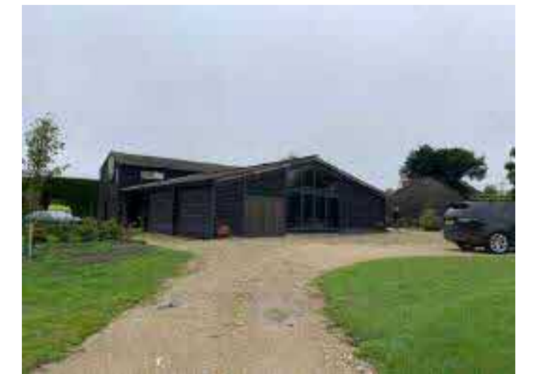
Existing Western Site Access - To be removed.
