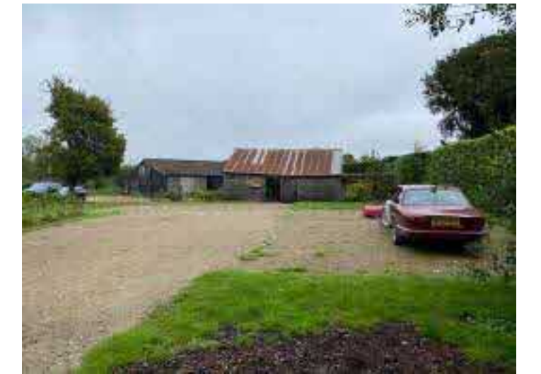
Existing Southern Site Access - To be retained.
