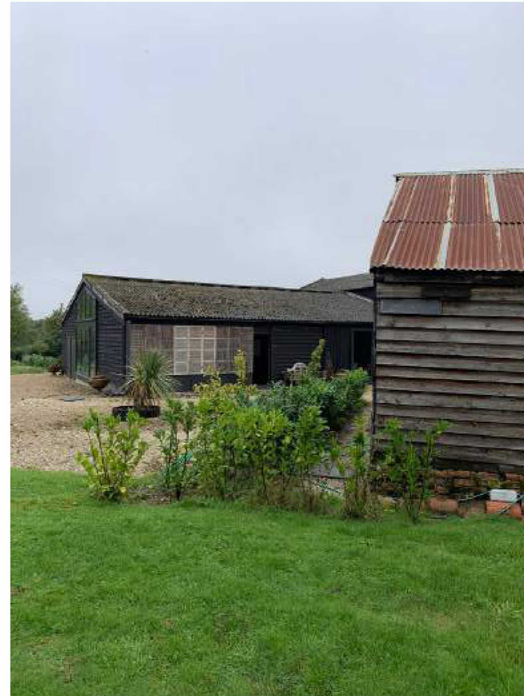
Outbuilding & Big Barn South Eastern Elevation:
