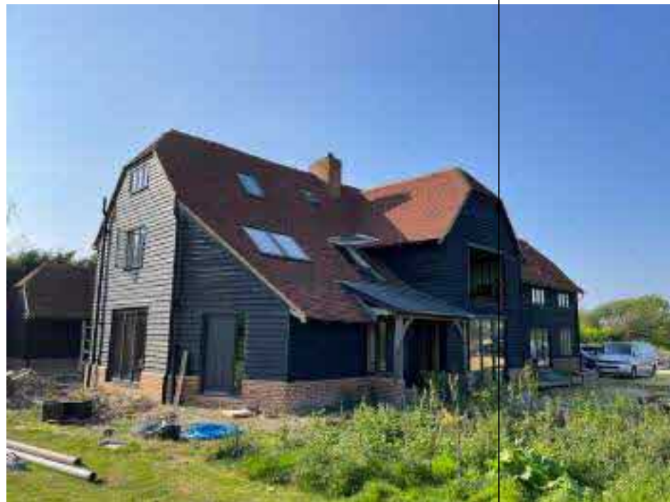
4. Converted traditional Essex Barn.
