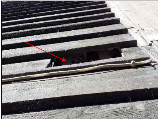
Photo 7. Gap in outer wall for ventilation Building 1
