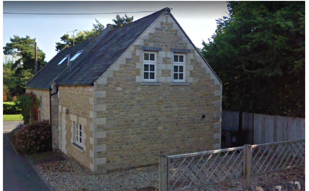
Extension recently built, property adjacent
