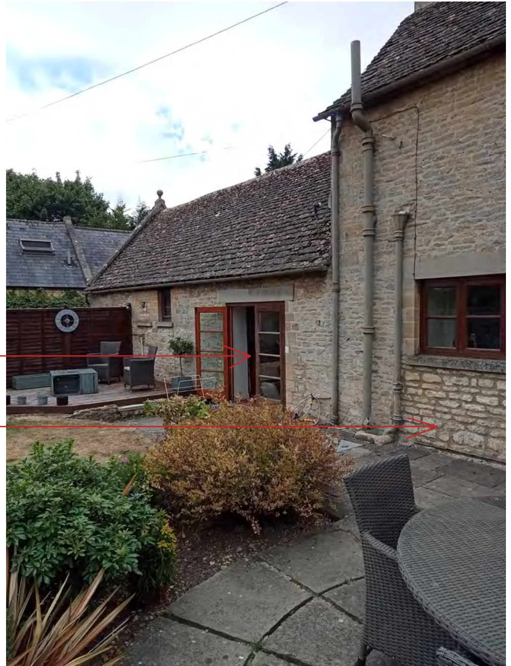
Photo barn roof
