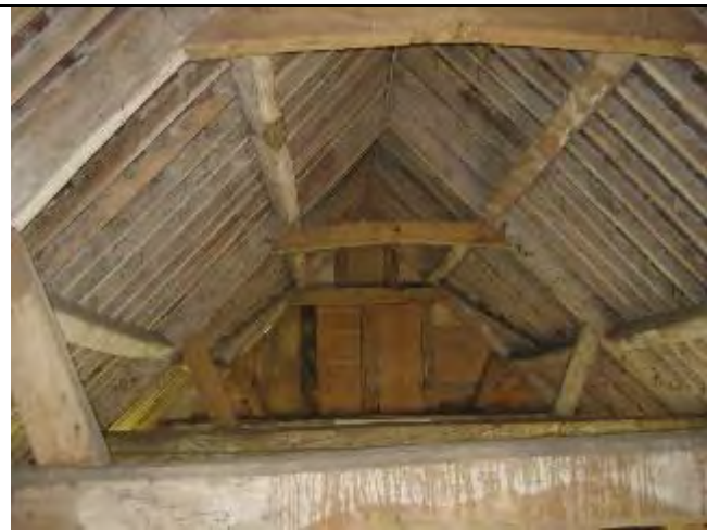
Interior of barn roof
