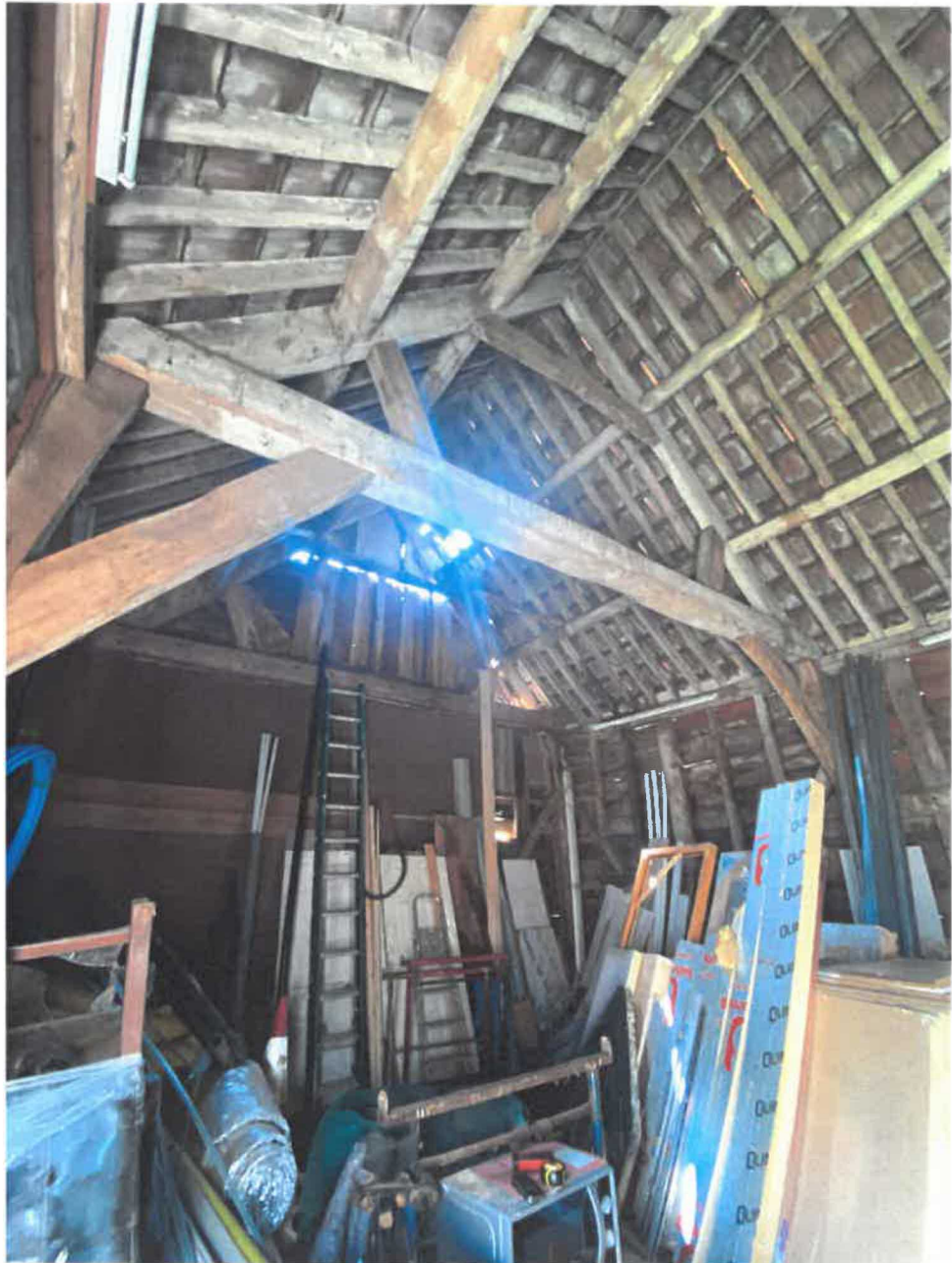
Roof truss with substantial knee bracing to maintain lateral stability
