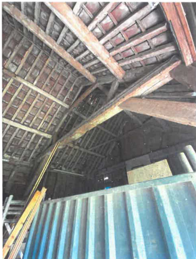
Another view on the substantial roof trusses and purlins
