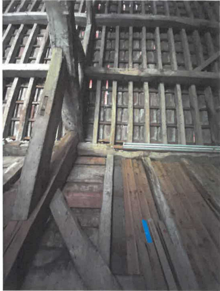
View on underside of roof within Barn, note substantial truss and purlins
