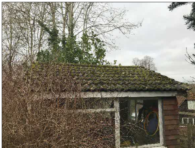
Plate 33. Side, eastern aspect, of the shed/summer house
