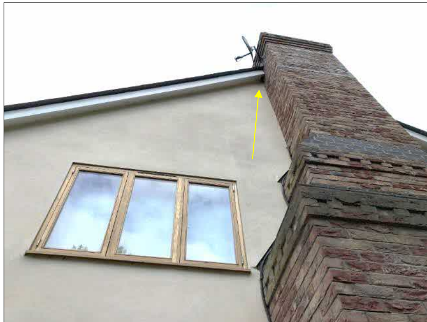
Plate 23. Example of gaps at weatherboarding, lead flashing and ridge tiles
