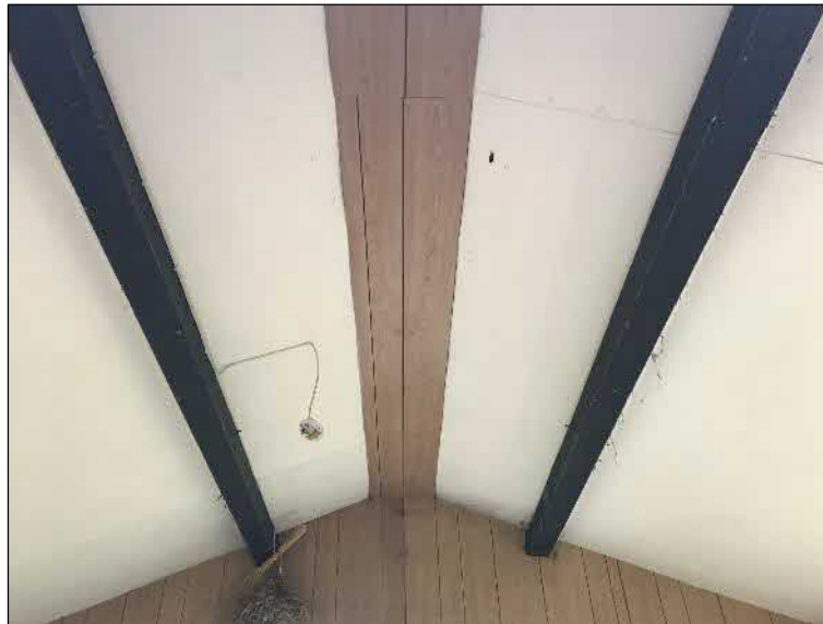
Plate 34. Internal of the shed/summer house
