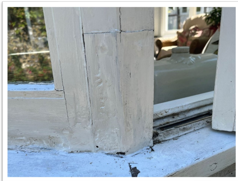
Image 11: Example of repair
