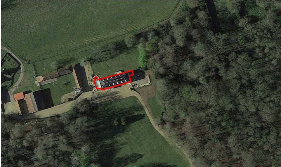
Figure 2. Location of the surveyed area. The footprint of the surveyed structure is shown by the red line.
