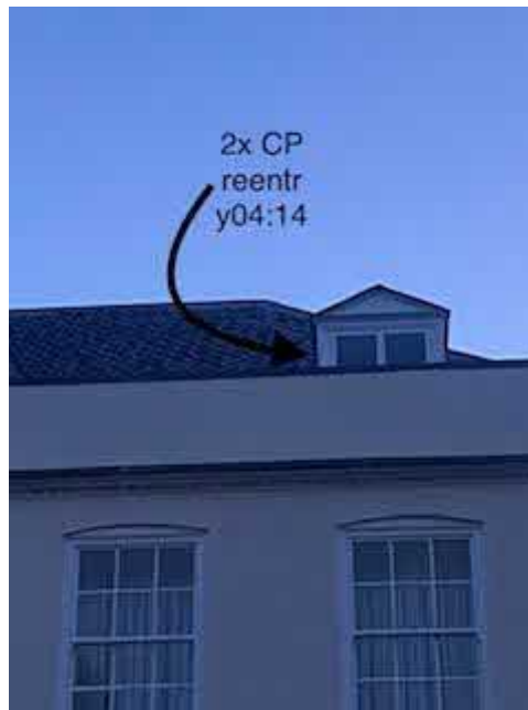
Image 5. Common Pipistrelle re-entry 26/05/22
