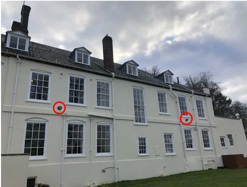
Image 3. The front face of the residential building, with the same features (eaves, walls and roofing) as the rest. Floodlights are highlighted.
