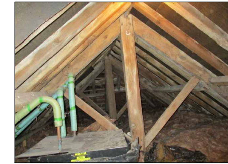
PHOTOGRAPH OF KINGPOST TRUSSES ARE AT 2.4 m CENTRES
