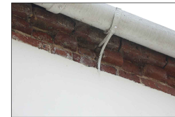
HALF ROUND CAST IRON GUTTER WITH METAL SUPPORT BRACKETS GROUTED INTO MASONRY
