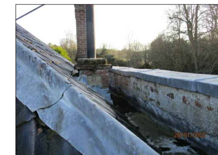
PARAPET WALL ON ROOF SIDE, CHIMNEY STACK AND LEAD LASHING
