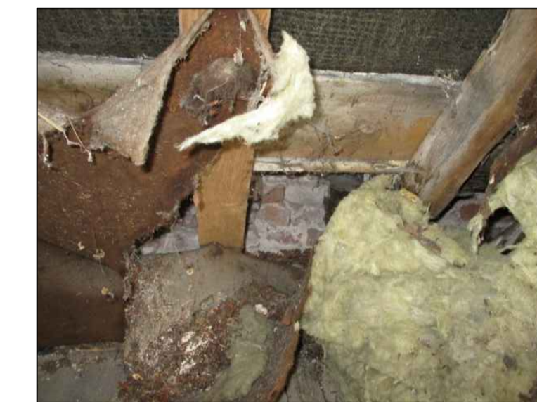
RAFTERS TOWARDS ROOF PLATE LEVEL
