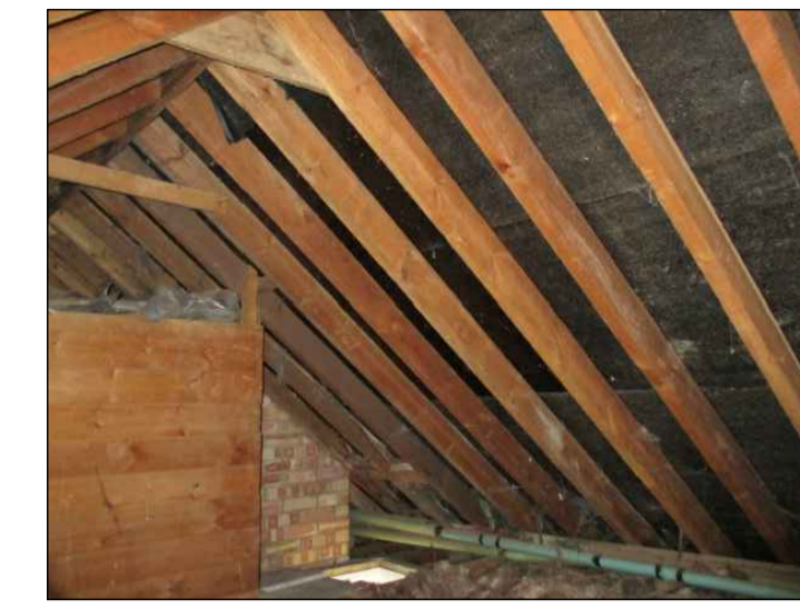
PHOTO THROUGH ACCESS TRAP ON 1 - 1
