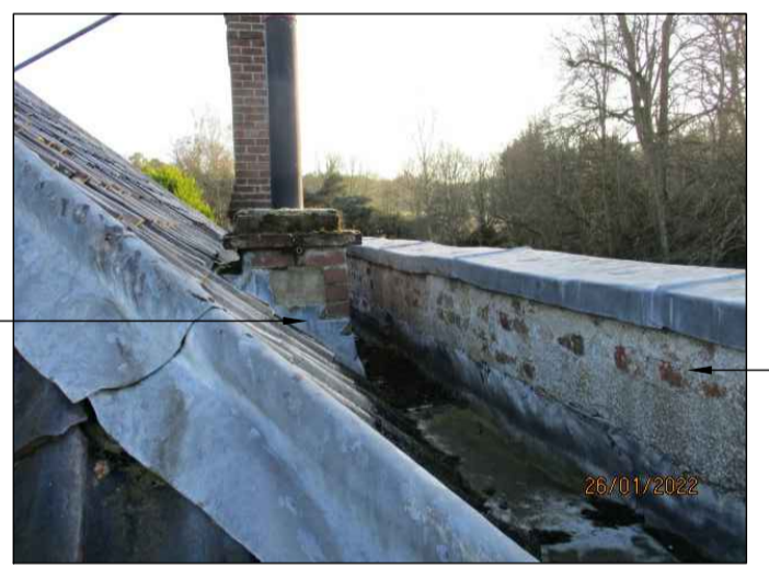
PARAPET WALL ON ROOF SIDE, CHIMNEY STACK AND LEAD LASHING
