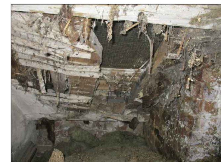
PHOTO TAKEN THROUGH ACCESS PANEL (WEST HIP)
