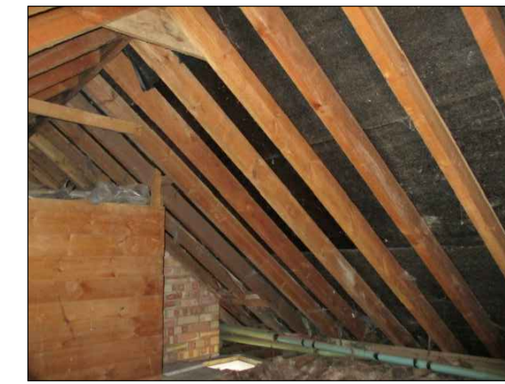
PHOTO THROUGH ACCESS TRAP ON 1 - 1
