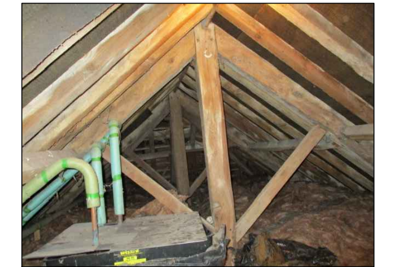
PHOTOGRAPH OF KINGPOST TRUSSES TRUSSES ARE AT 2.4 m CENTRES
