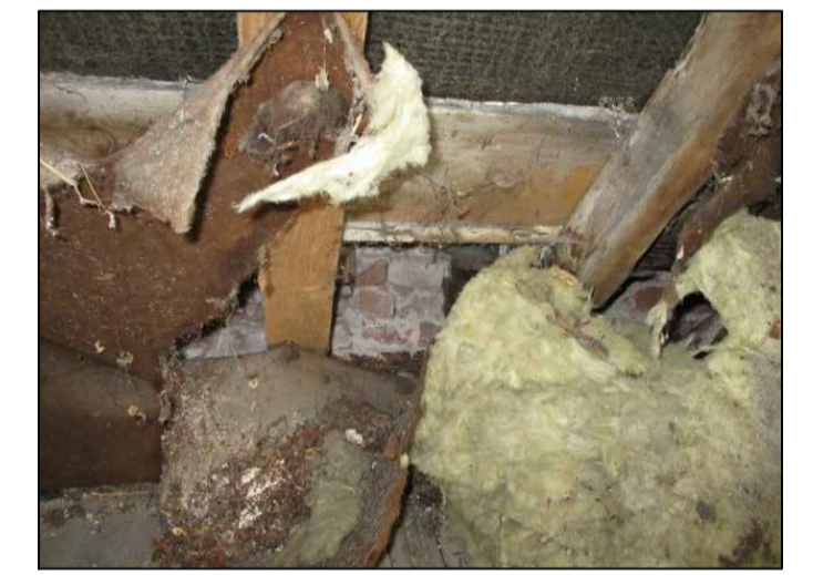
RAFTERS TOWARDS ROOF PLATE LEVEL
