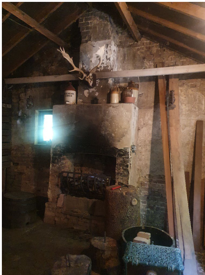
Photograph 6 – Inglenook fireplace with exposed brickwork to be retained.
