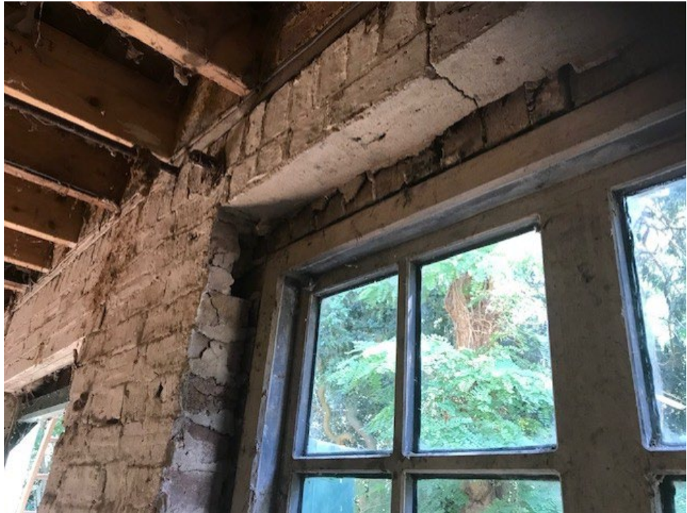
Photograph 2 - Example of existing windows set forward within the reveal, flush to the window to be replaced with windows which are set back within the reveal.
