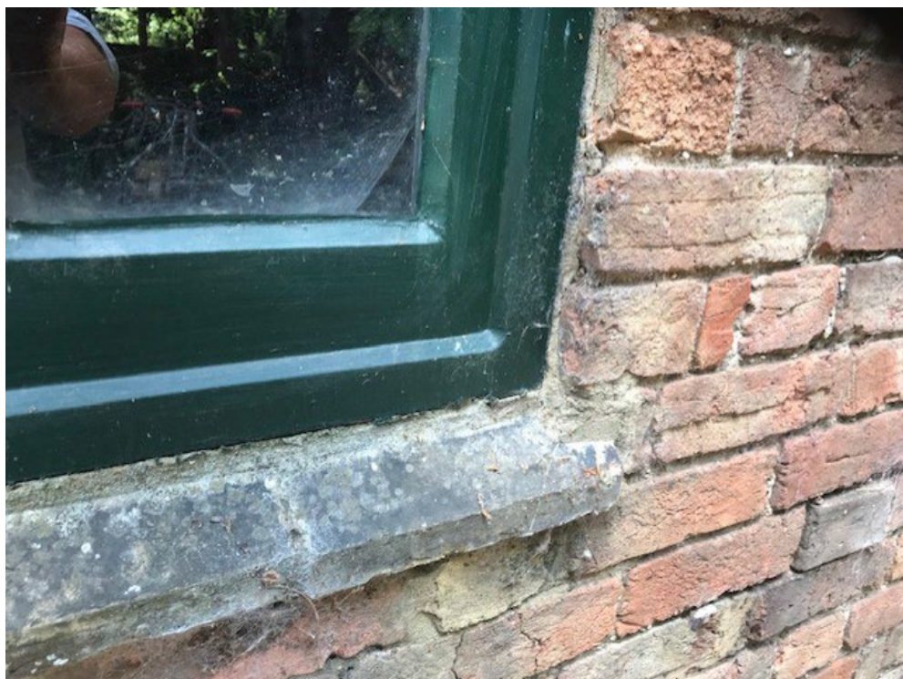
Photograph 3 - Example of existing windows set forward within the reveal, flush to the window to be replaced with windows set back within the reveal.
