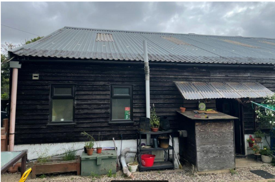
Partial side elevation of building showing The Flat access.
