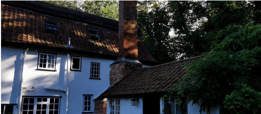
The Main House and Outbuilding to be Converted
