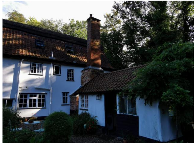
P4: B 2 West Elevation showing lifted tiles
