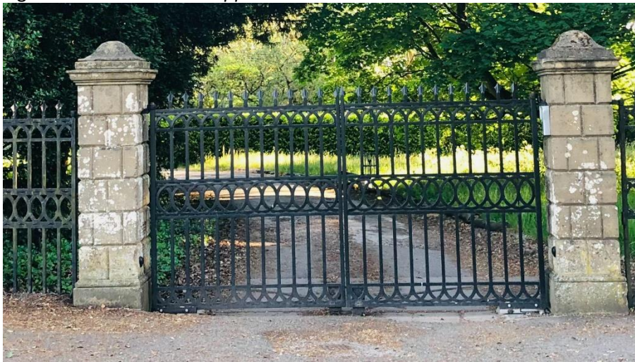
Fig 3. Gates installed at Papplewick Hall
