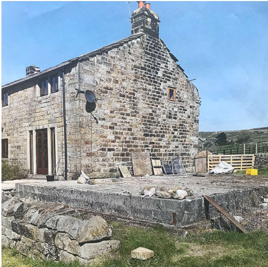
Image 1- Existing South facing gable end, Carrs Fam, Rowland Lane, Hebden Bridge
