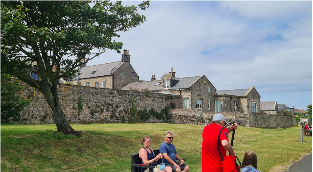
Figure 16. View from the south-west promenade on the Castle Green westwards. 6 The Wynding is the dominant form with two gables and a south-facing gable dormer.
