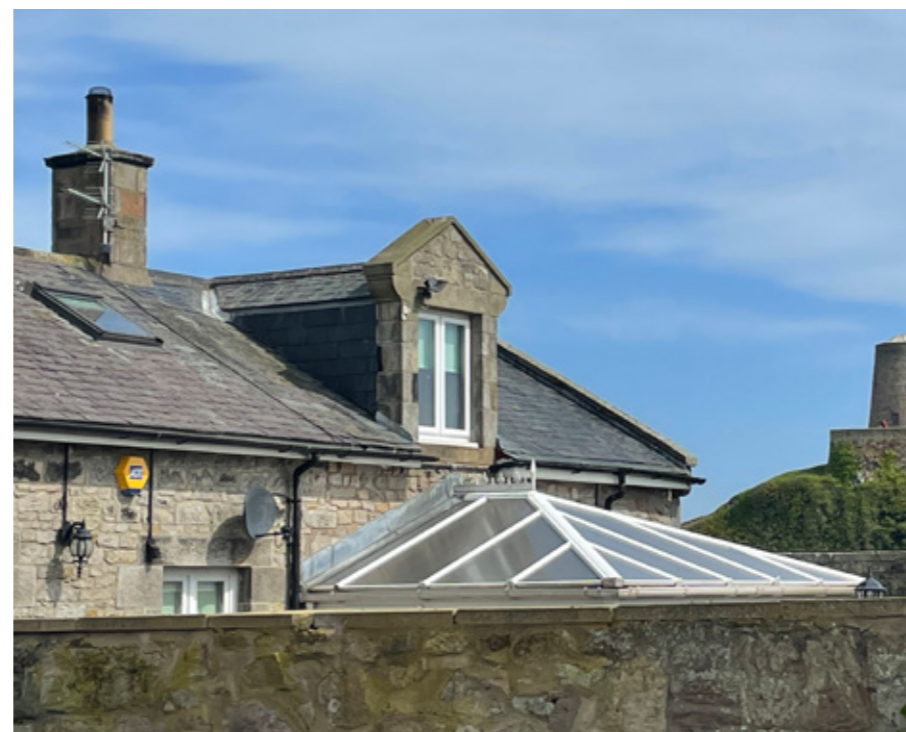
Figure 52. Stone dormer with lead cheek walls.
