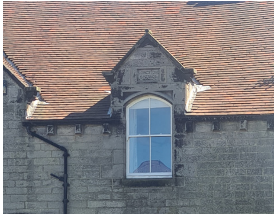
Figure 49. Stone dormer with slate roof.
