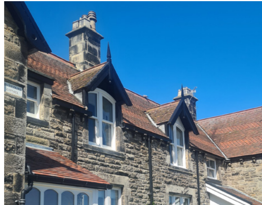
Figure 50. Victorian timber dormer with lead cheek walls and clay roof.
