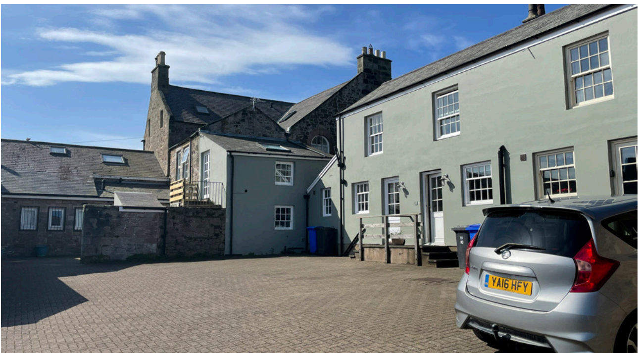
Figure 28. Rear elevation of the Wynding House and neighbouring properties.
