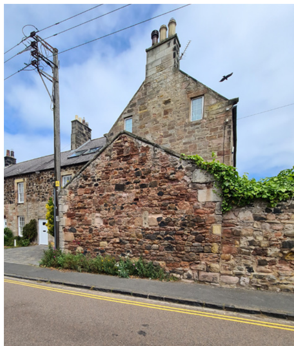
Figure 30. West gable of the House.
