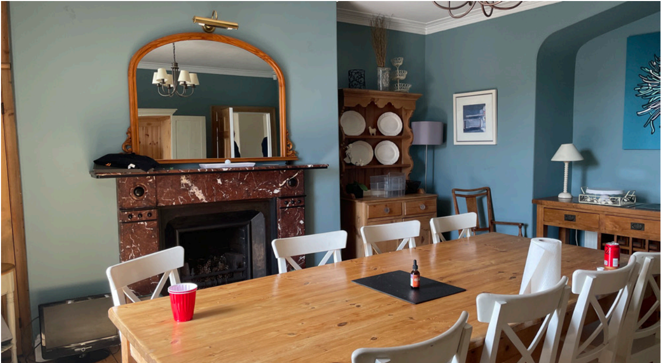
Figure 22. The chimney in the dining room has been altered in size with a fireplace not original to the house.
