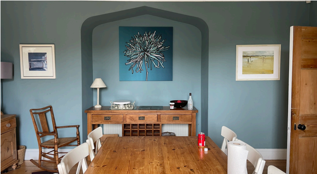
Figure 25. The blocked off opening between the dining room of the Wynding House and the living room of 4A The Wynding.
