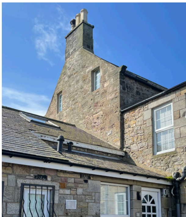
Image 29. East gable of the House.
