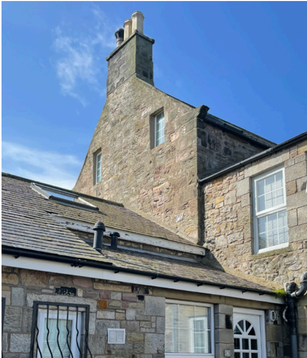
Image 9. East gable of the House.
