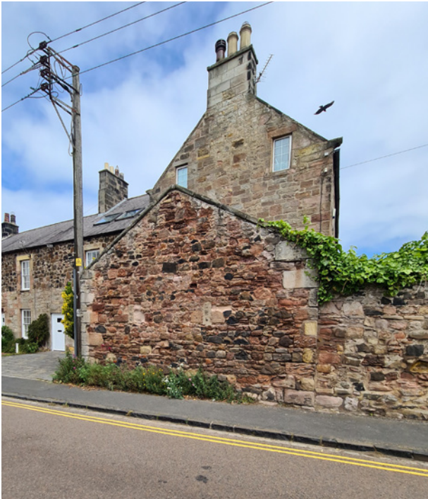
Figure 8. West gable of the House.
