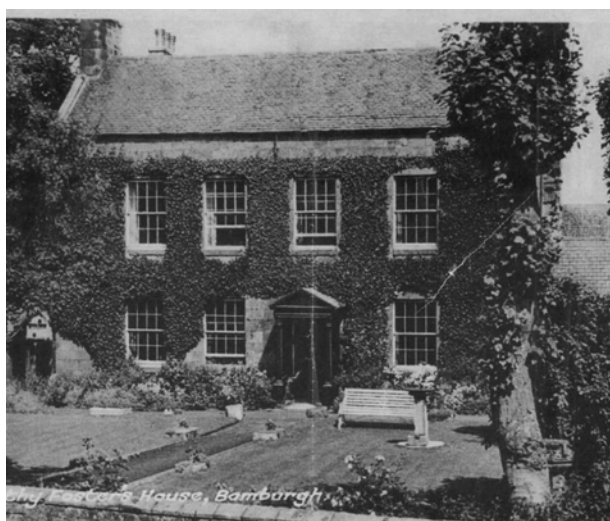
Figure 27. Comparison of window arrangements between the historic, likely original, arrangement and current, likely late Victorian or Edwardian, arrangement.
