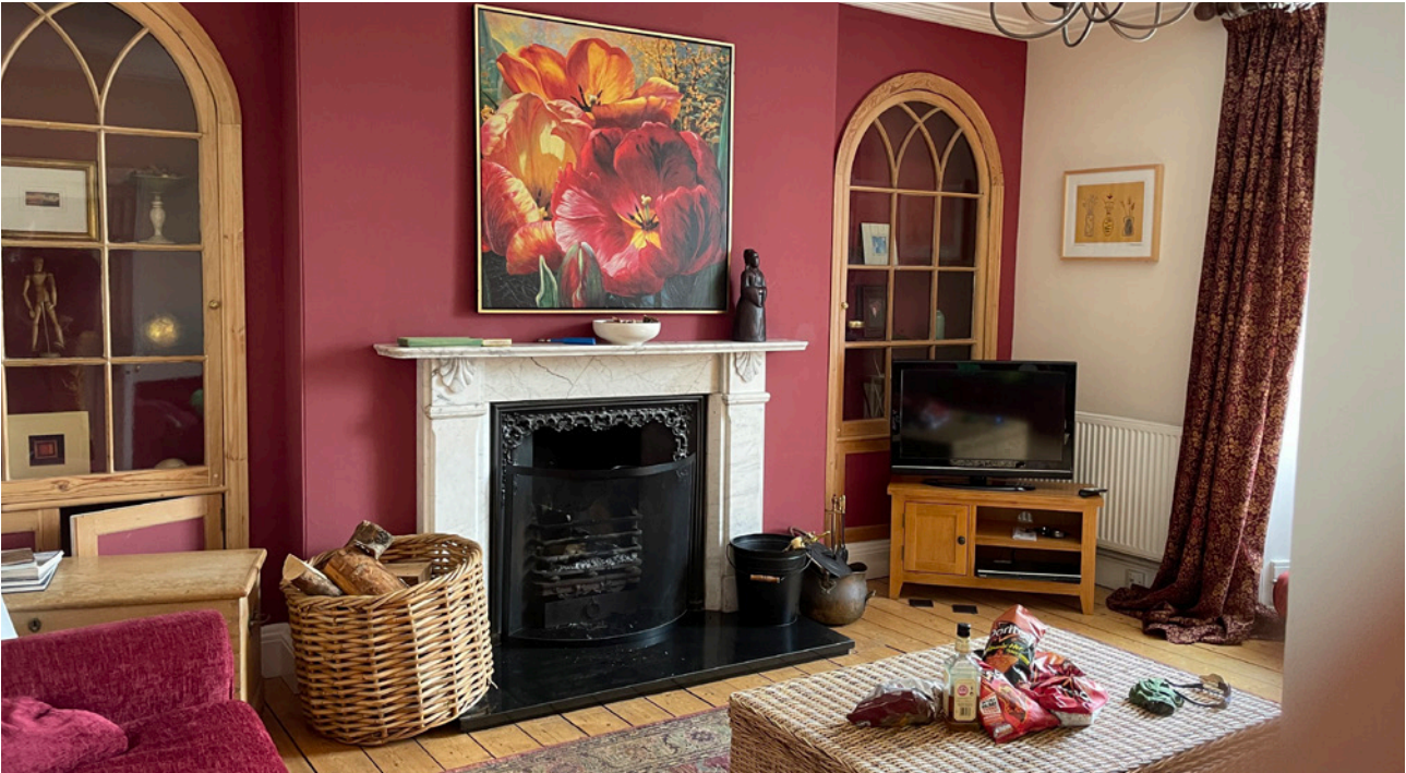
Figure 23. The chimney in the living room is unaltered with Victorian cabinets built-in to the sides.
