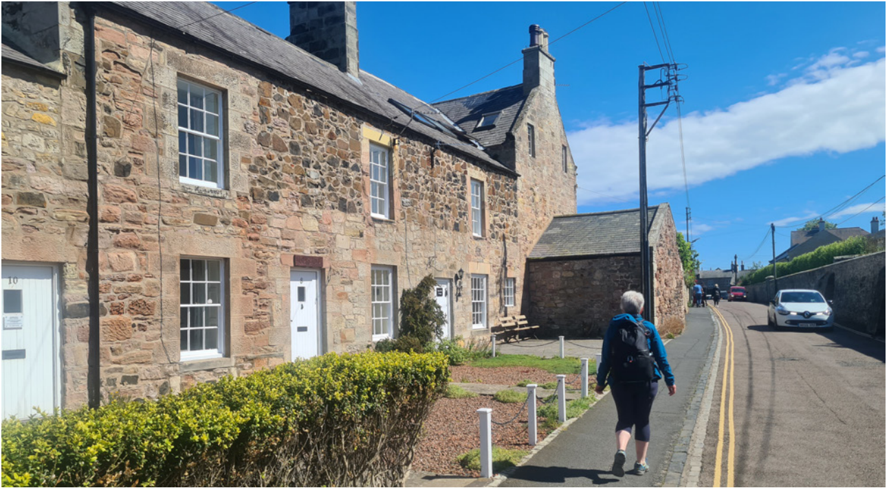
Figure 5. View along the Wynding southward, showing the change of scale of the rear of the main house.
