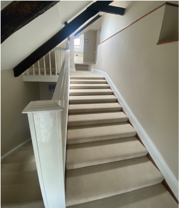
Figure 24. The staircase between the first floor and the roof space (now second floor) was introduced with uncomfortable low risers and long goings, likely due to the height constraints with heights of the beams being very low.
