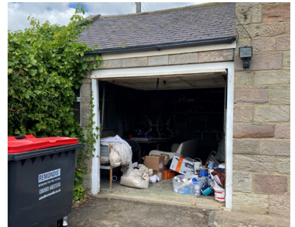
Fig 38. The existing garage utilised as storage space..
