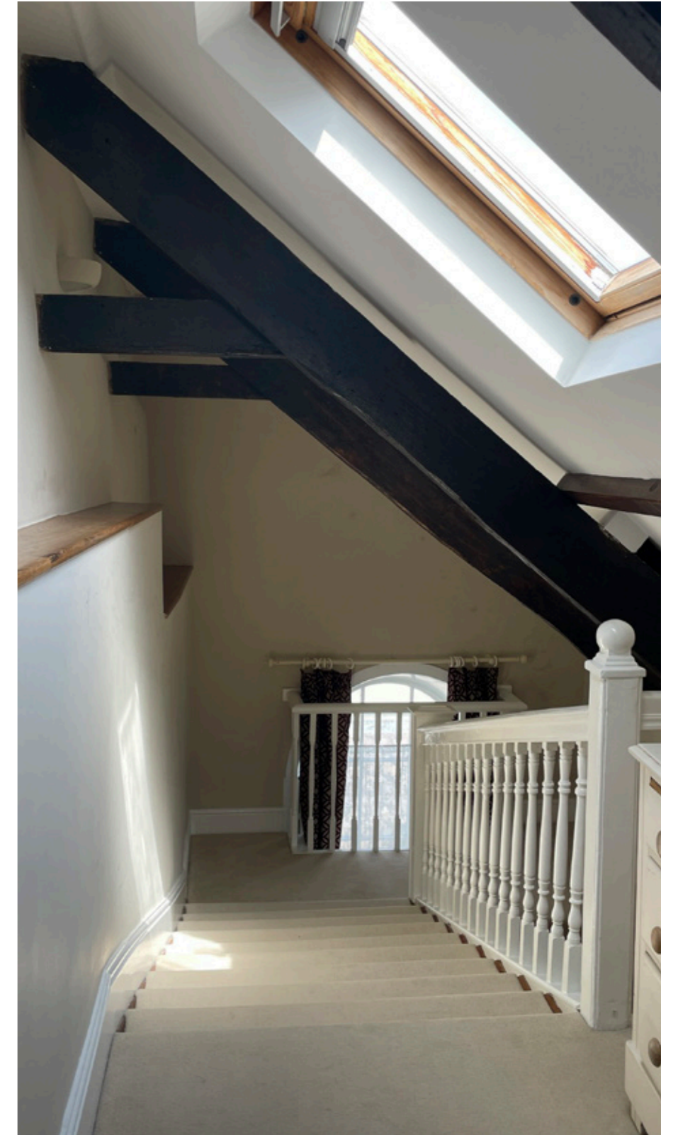
Fig 41. The staircase between the first floor and the roof space (now second floor) was introduced with uncomfortable low risers and long goings, likely due to the height constraints with heights of the beams being very low.
