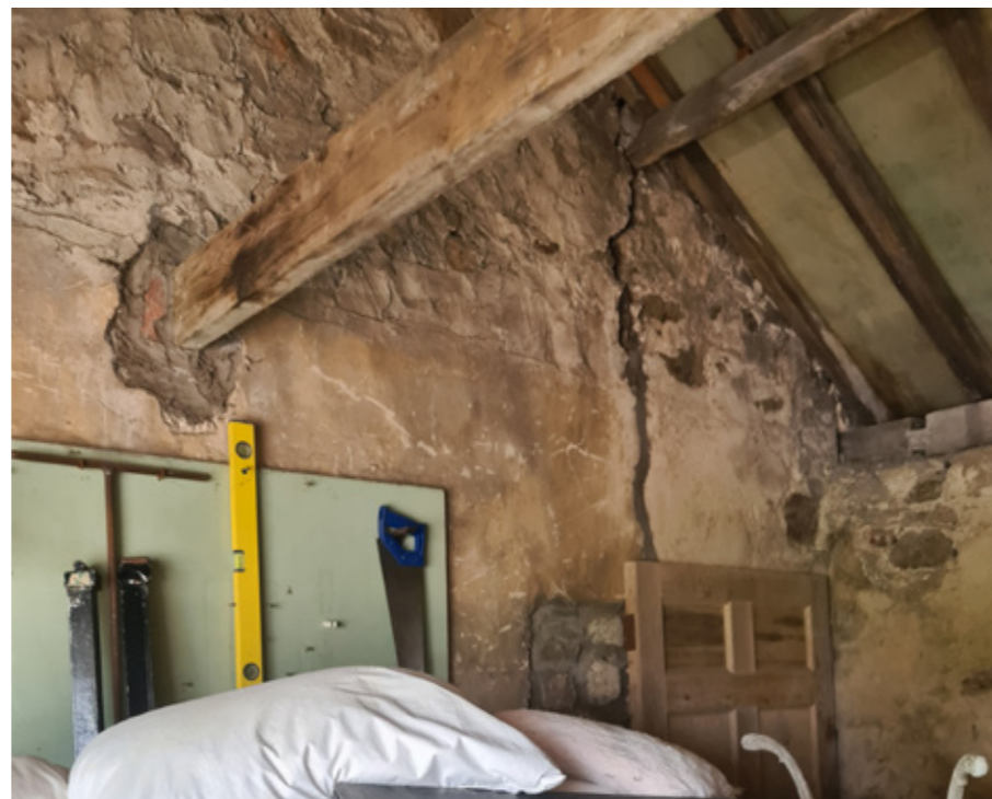
Fig 37. The existing exposed roof trusses in the garage
