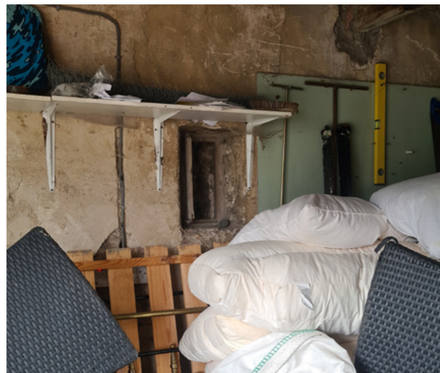
Fig 29. Infilled arrow slit windows to be reinstated - Internal view.
