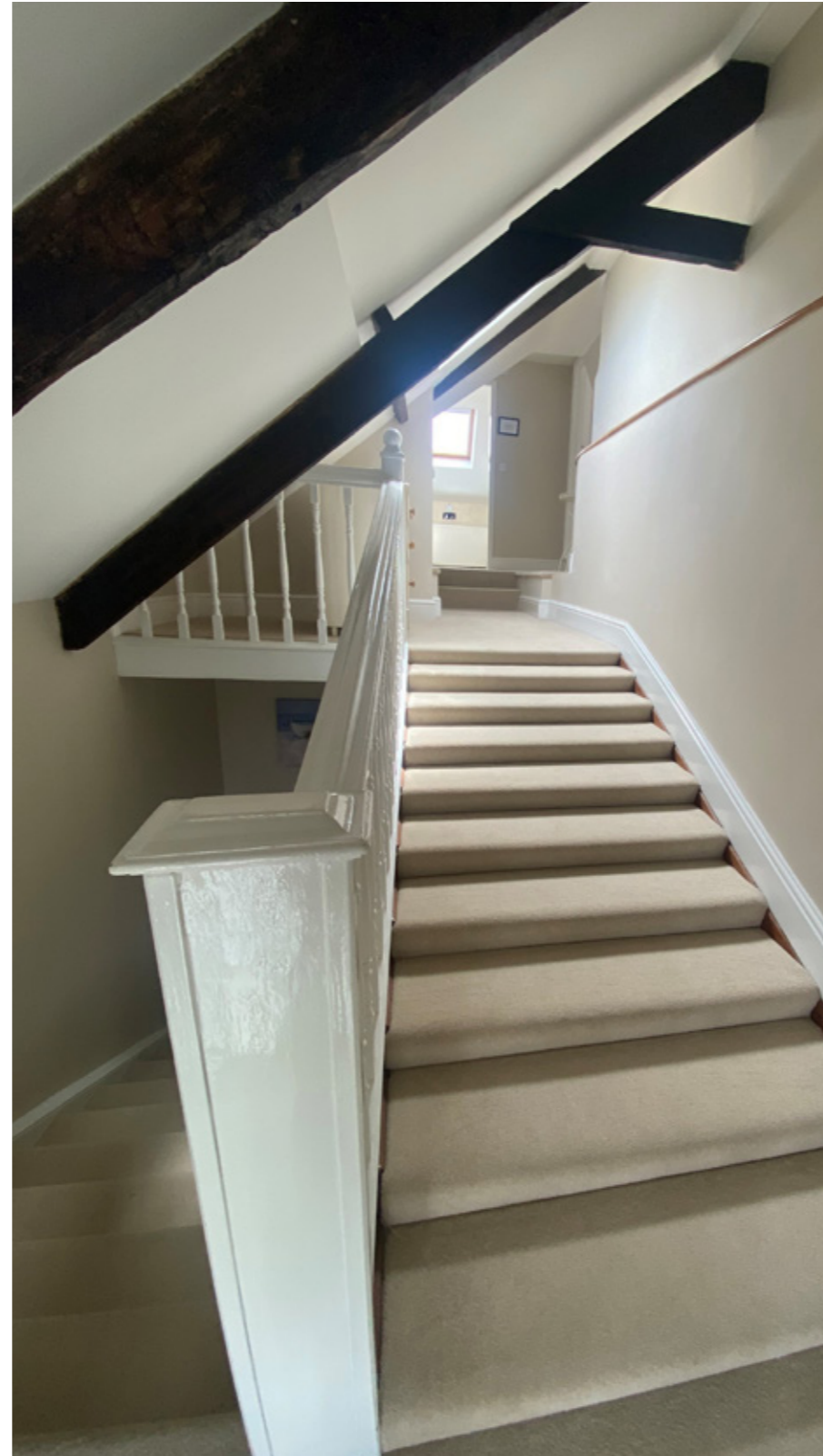
Fig 41. The staircase between the first floor and the roof space (now second floor) was introduced with uncomfortable low risers and long goings, likely due to the height constraints with heights of the beams being very low.
