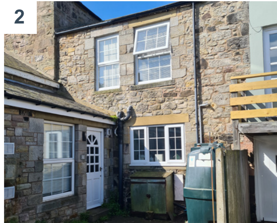
Replacement of inappropriate later additions
