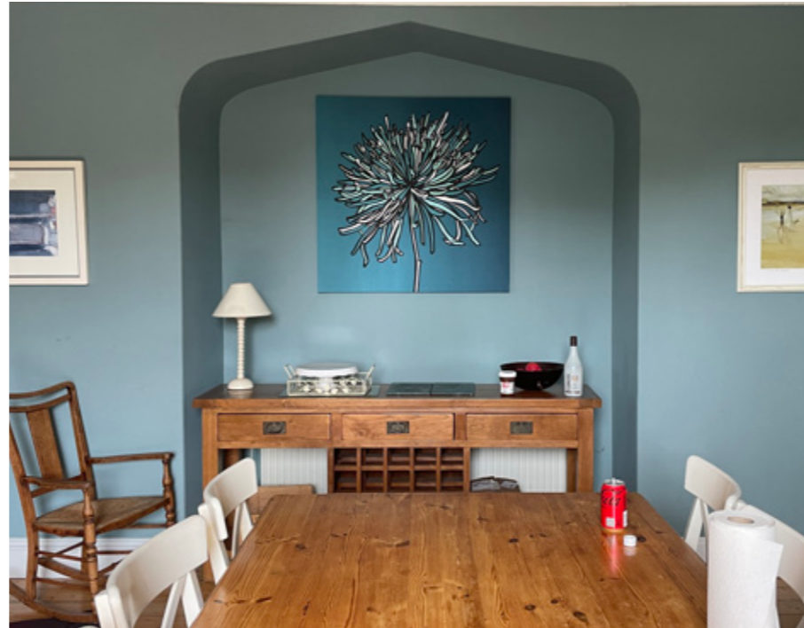
Fig 35. The blocked off opening between the dining room of the Wynding House and the living room of 4A The Wynding.
