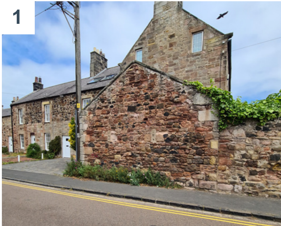
Repairs to the stonework and slate
