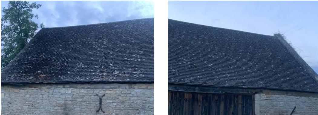
Figs. 7 & 8 Ridge and roof tiles to the east
