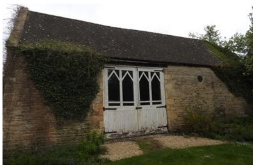
Fig. 1 West facing aspect of the barn
