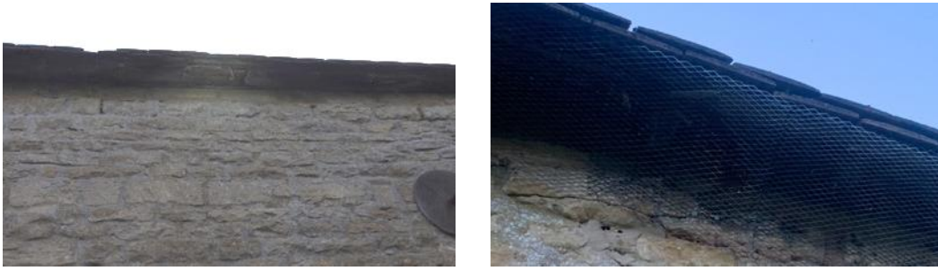
Figs. 11 & 12 Sealed eaves to the west (L) and east (R)
