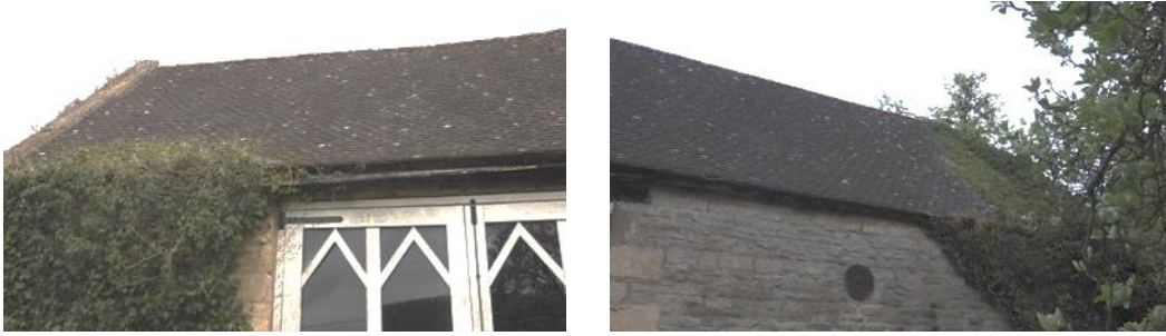
Figs. 5 & 6 Ridges and roof tiles to the west
