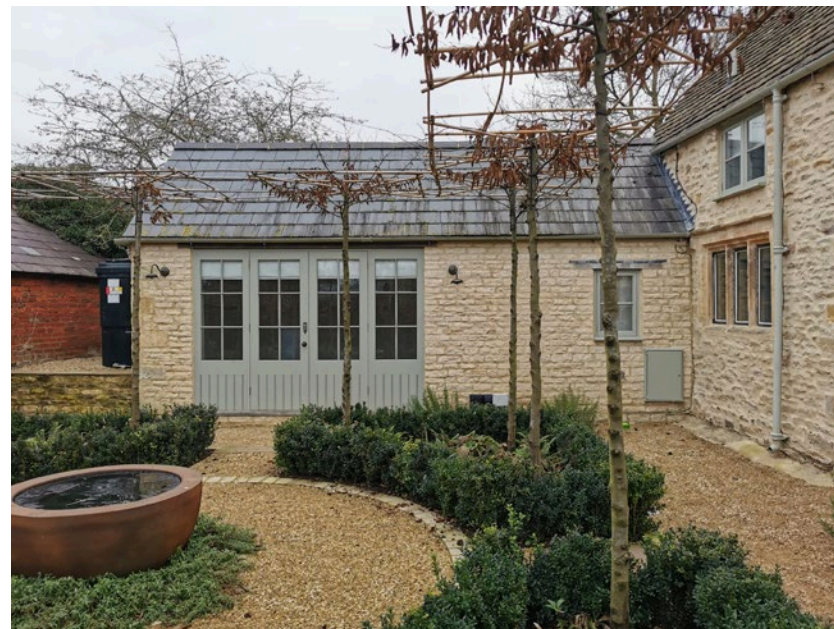
Existing landscaped courtyard and doorset
