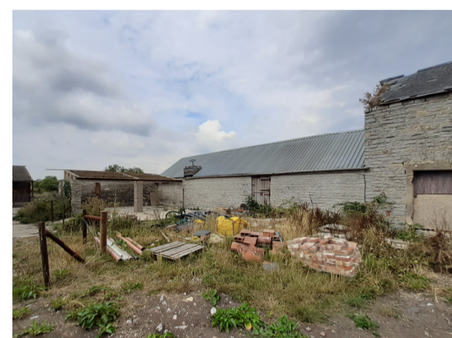
Site Photo 01. Existing West elevation of Barn viewed from side yard.
