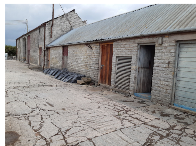
Site Photo 03. Existing East elevations of Barn viewed from top yard.
