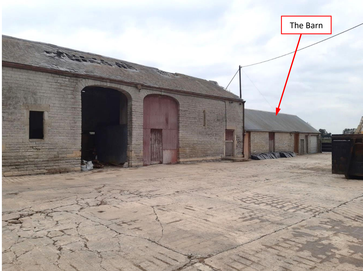
Image 3 – Western two-story and single-storey barns viewed from courtyard.
