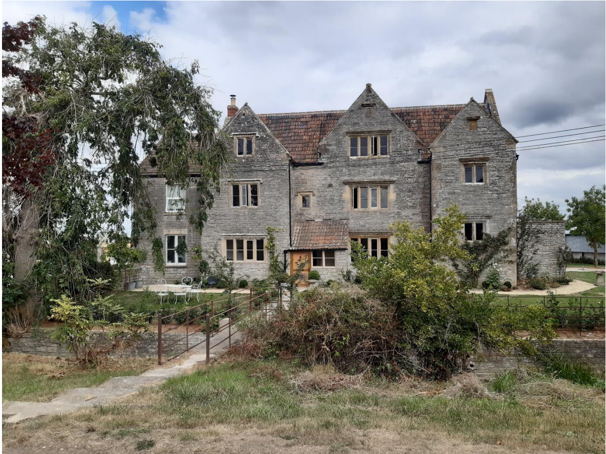
Image 1 – Front (south) elevation of Manor Farmhouse viewed from the Kennard Moor Drive.
