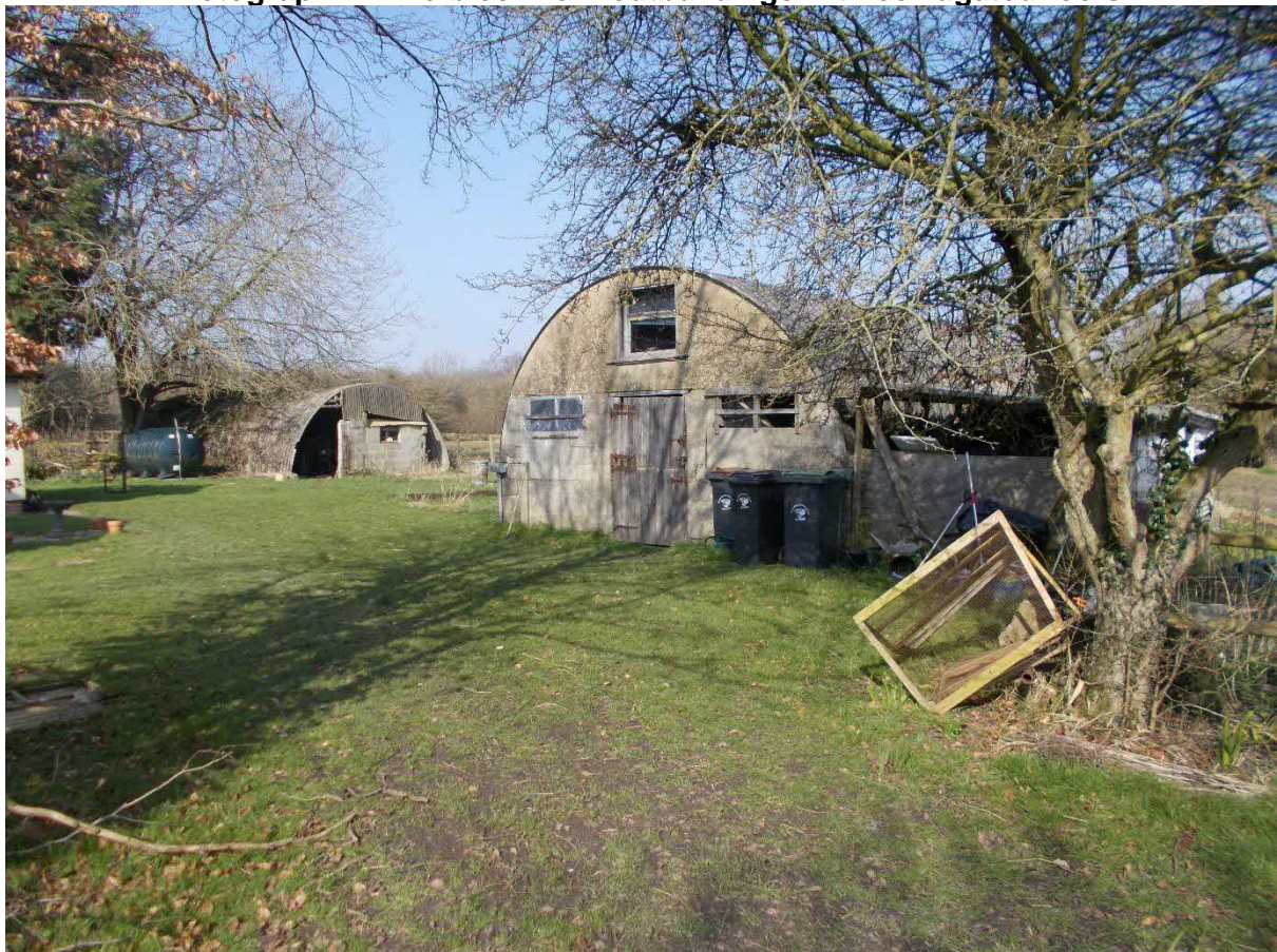
Photograph 4: Two blockwork outbuildings with corrugated roofs
