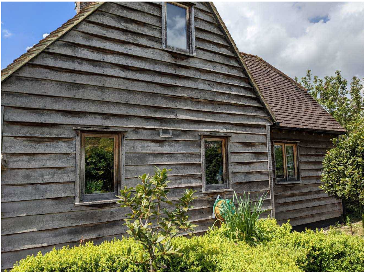
2003 extension from east
