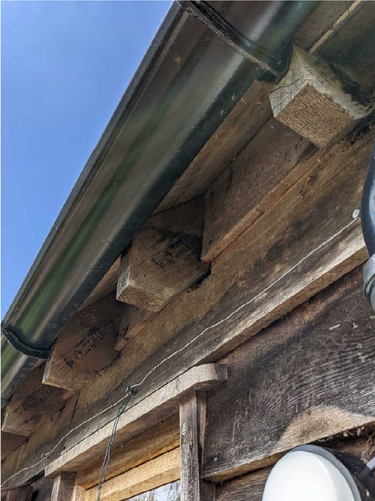
Softwood rafter feet/ends and oak boarding
