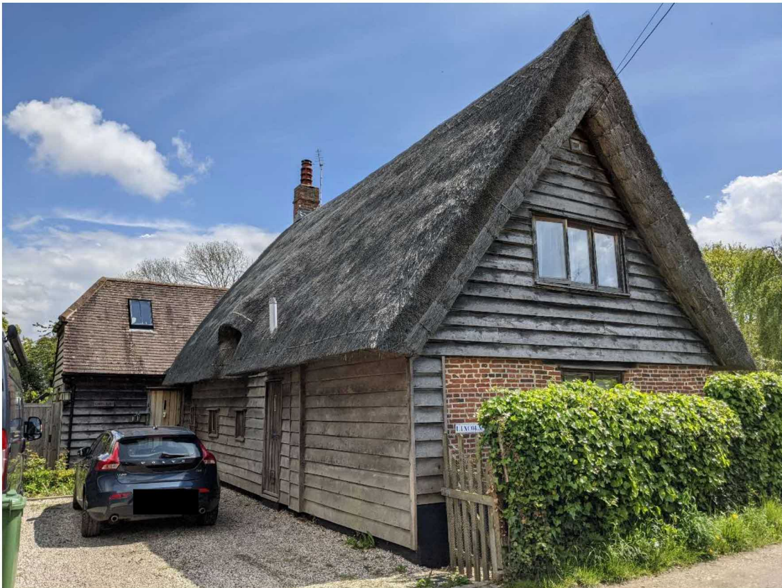
Driveway and front door approaches from west
