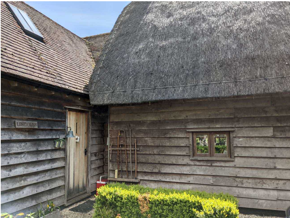
Junction of historic cottage and earlier extension
