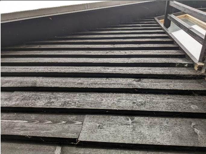
Photo 3 Tight fitting boards on south gable of cart lodge
