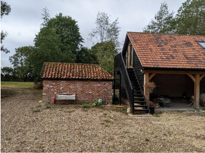
Photo 1 East elevation of outbuilding and cart lodge
