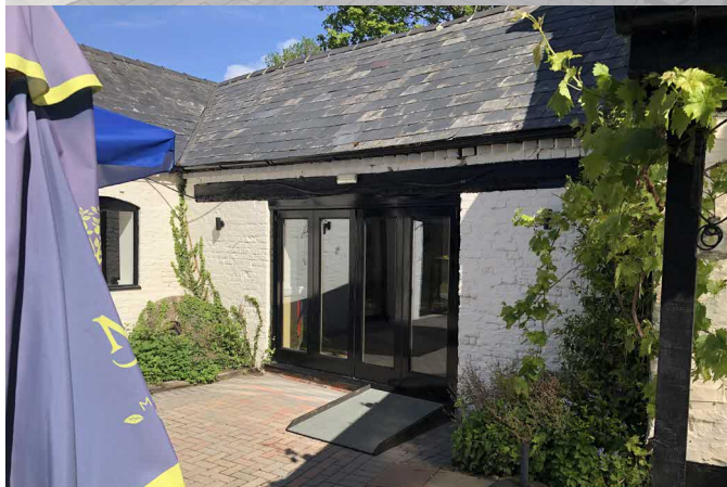
East leg of existing function room
