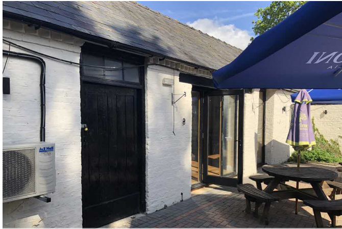
Door to the bar and glazed screen to function room
