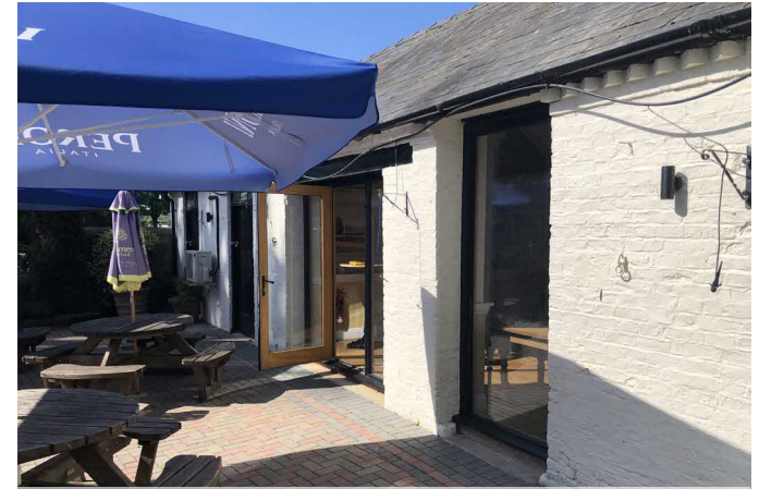
Full height window to be replaced with door
