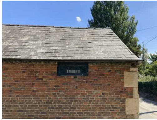
Photograph 2: West building aspect.
