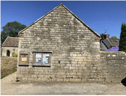
Photographs 1: South building aspect.
