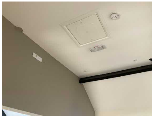
Photograph 6: Loft access hatch.
