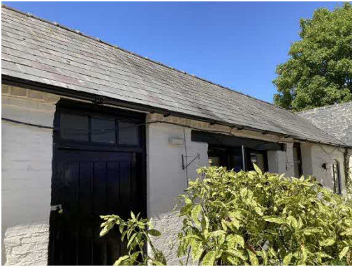
Photograph 3: East building aspect.
