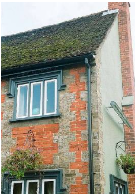
Examples of brick types and brick detailing, flint walls with brick detailing (images from Conservation Area Appraisal)
