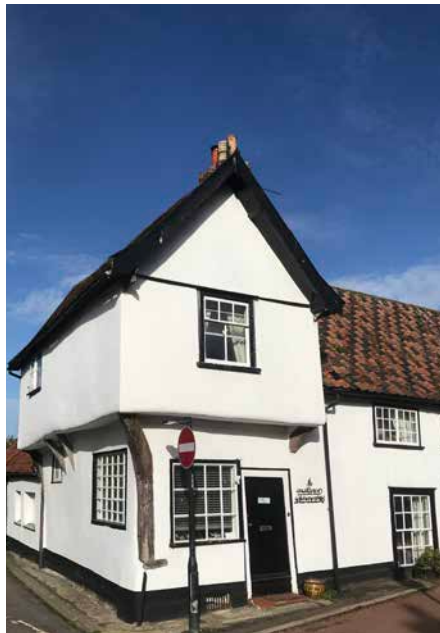
Example of jettied first floor, patterned roof tiling
