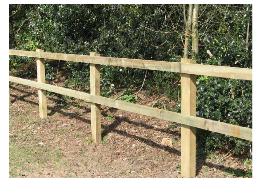
TIMBER POST AND RAIL FENCING
