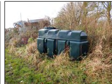
Photo 36 Empty Bunded 2,500L Oil Tank to West of Site, View South West
