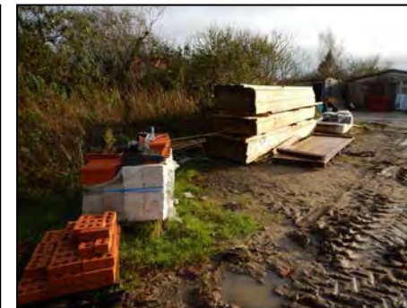
Photo 44 Storage in North West of Site, View East
