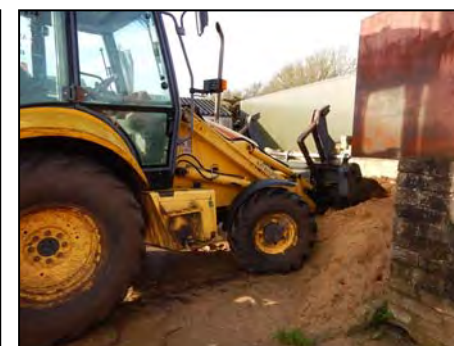
Photo 48 Machinery & Aggregate Storage South of Diesel Tanks, View West
