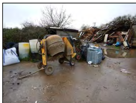
Photo 6 Cement Mixer & Storage, View South
