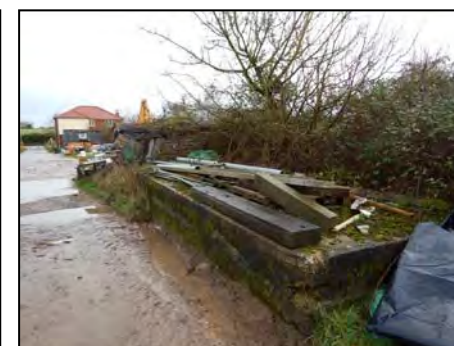
Photo 16 Material Storage on Site, View South West
