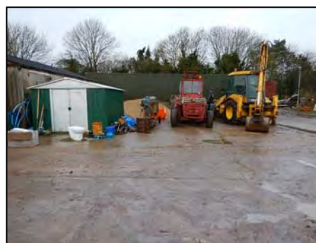
Photo 7 Machinery & Aggregate Storage in North of Site, View West
