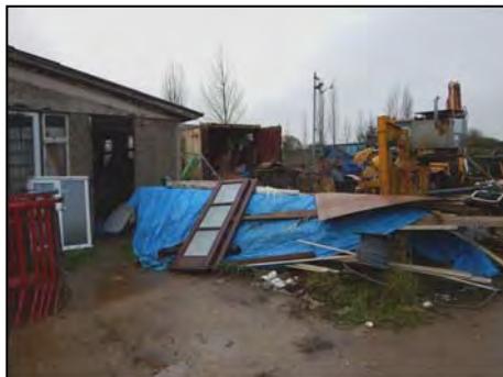
Photo 1 Storage to North East of Site, View South East
