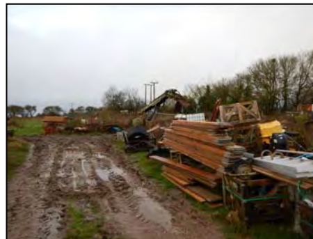
Photo 19 Material Storage in Centre of Site, View South West
