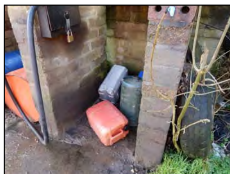
Photo 46 Fuel Containers Beneath Tanks in North of Site
