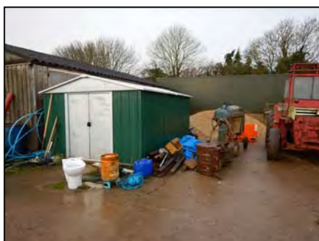
Photo 13 Building Equipment & Material Storage in North of Site, View West
