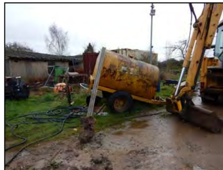
Photo 3 Machinery in North of Site, View South
