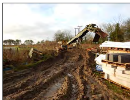
Photo 31 South West of Site, View South West
